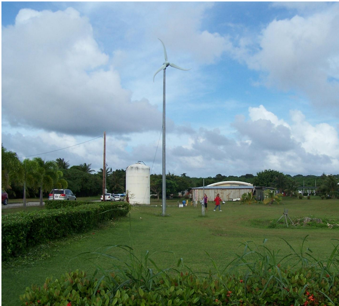
Figure 2. Skystream 2.4 kW wind turbine
