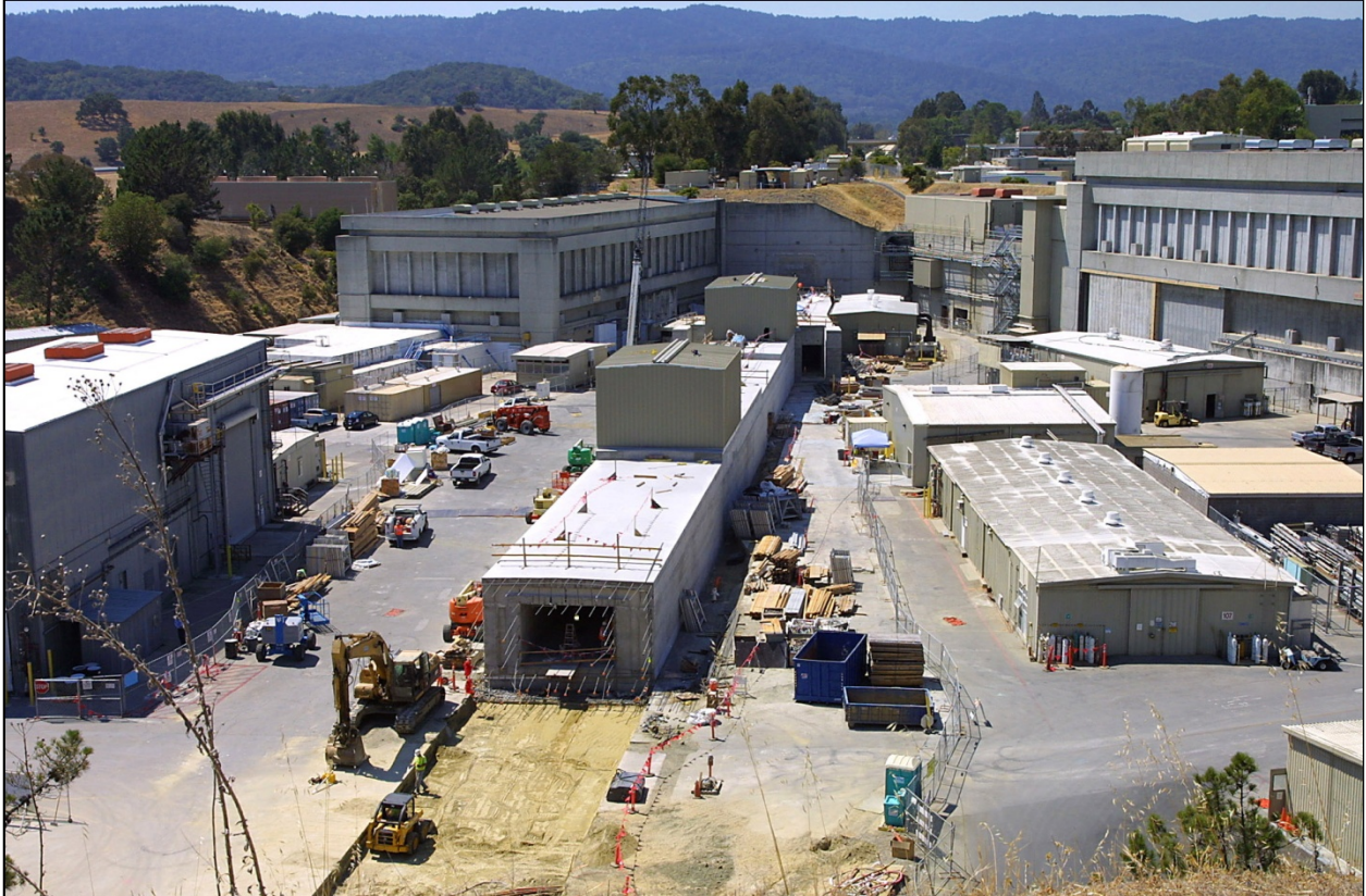
Photo A-1: Construction of the LCLS Beam Transport Hall across the SLAC Research Yard
