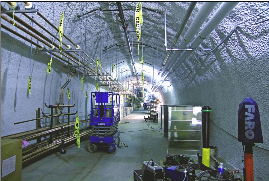
Photo A-2: Construction of the LCLS-I Undulator X-Ray Transport
