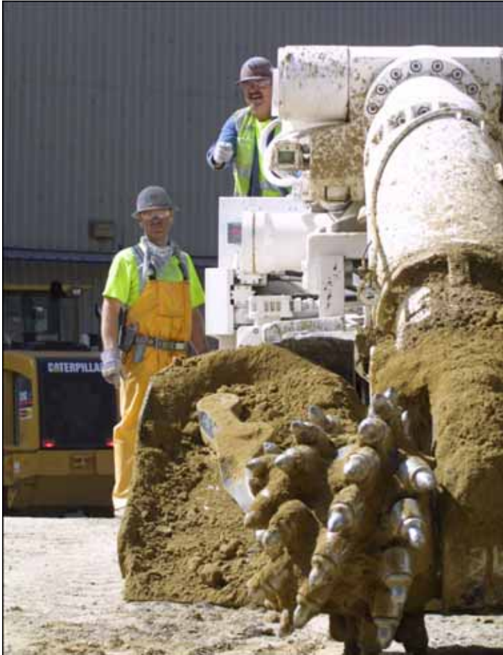
Figure 2-5 Road Header Used for Tunneling
