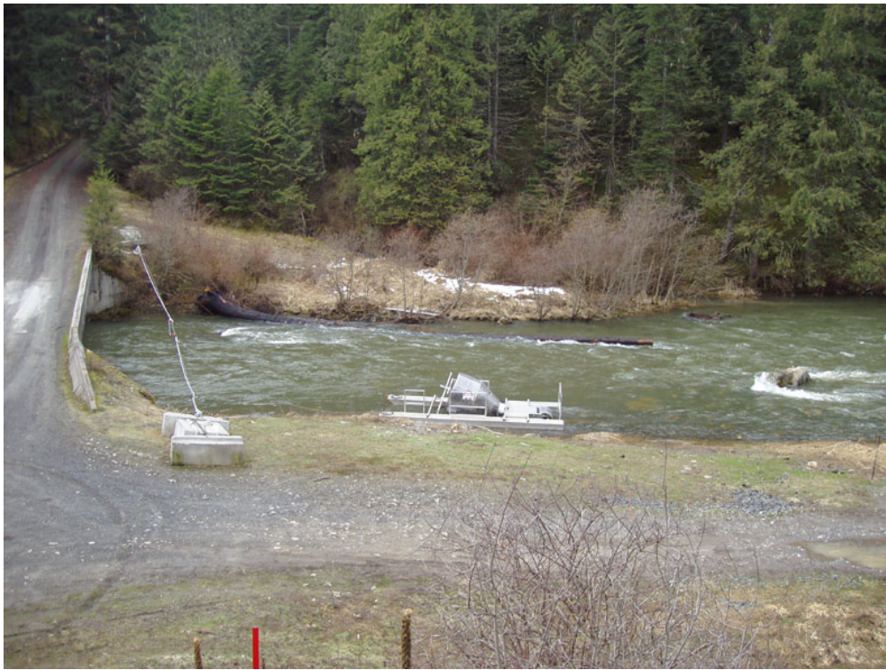
Photo 11. Looking South, View of Lolo Creek Road Bridge and downstream north/south bank from Lolo Creek Road from the north, June 211.
