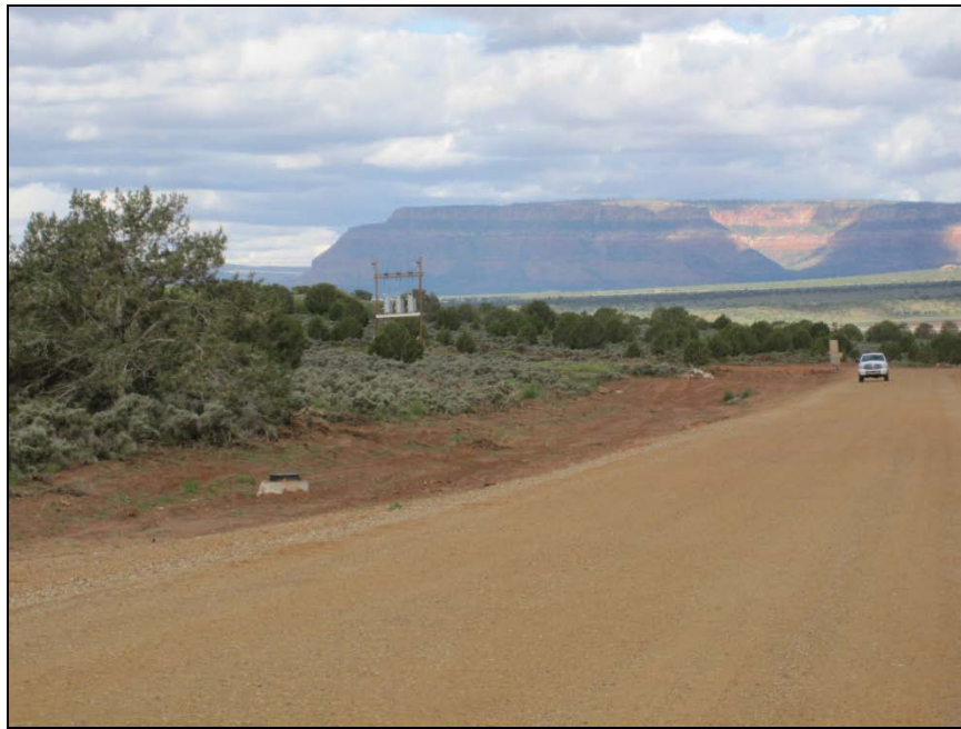
Figure 3-11. Sanitary Sewer on Kaneplex Road at Proposed Pilot Plant Site (recently installed to serve Public Safety Facility)
