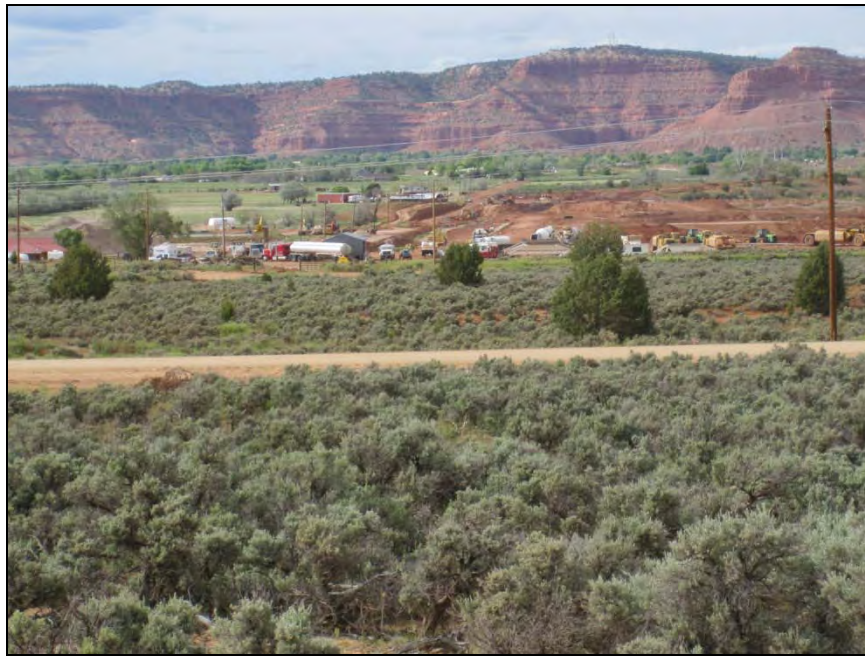
Figure 3-5. Telephoto View of Jackson Flat Water Supply Storage Project Construction from Proposed Pilot Plant Site
