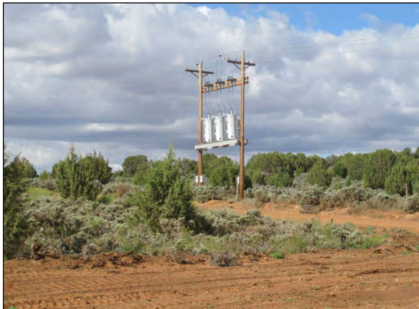
Figure 3-12. Transformer Substation on Old Landfill Road adjacent to Proposed Pilot Plant Site
