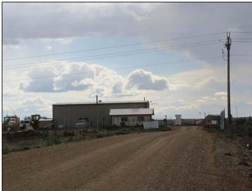
Figure 3-2. Kane County Landfill (east end of Kaneplex Road)
