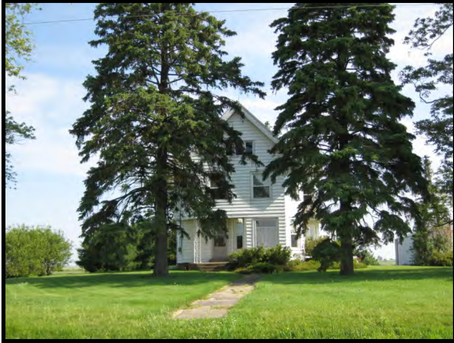
Photo 1 – Architectural Resource A1, south elevation.
