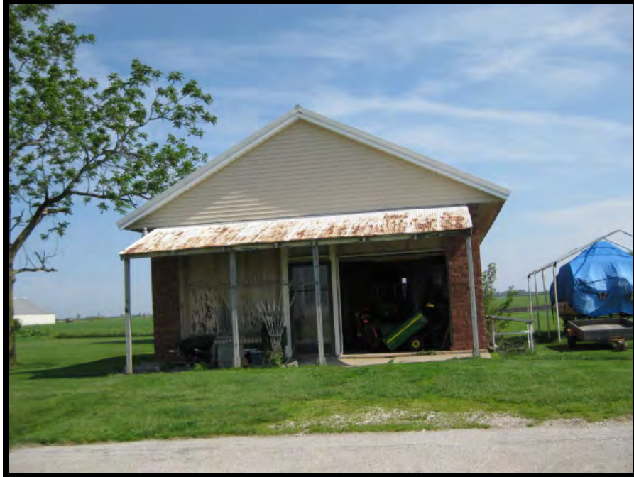
Photo 3 – Architectural Resource A2, south elevation.
