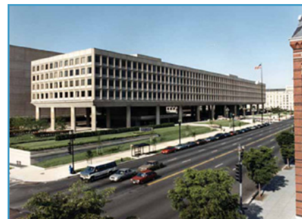
DOE Headquarters Forrester Building in Washington, D.C.
