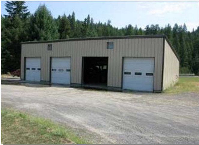
View 6. Klickitat Hatchery Site: Storage building within the Klickitat Hatchery Complex looking west.
