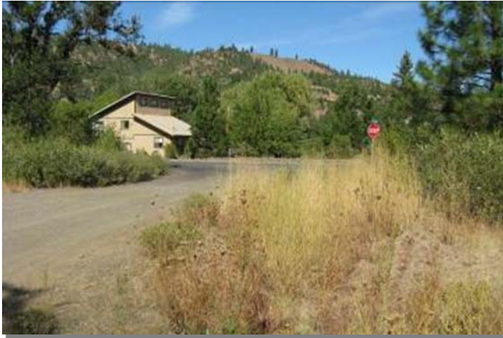
View 1. Wahkiacus Hatchery Site: Intersection of Klickitat Trail and Schilling Road, looking north at the office/residence structure.
