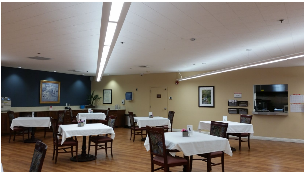
Figure 12. Dining room with direct/indirect LED lighting. Although dimmable, it was fixed at 4100 K and was used at full output for mealtimes.
