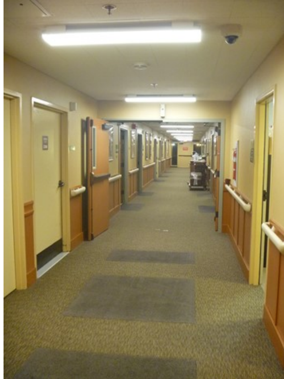
Figure 6. Photo of typical resident-room corridor, with LED color-tunable overhead lighting installed. Daytime setting with 4100 K color temperature and maximum light output is shown here, reflecting the fixed output setting intended to mimic the original undimmable fluorescent lighting.
