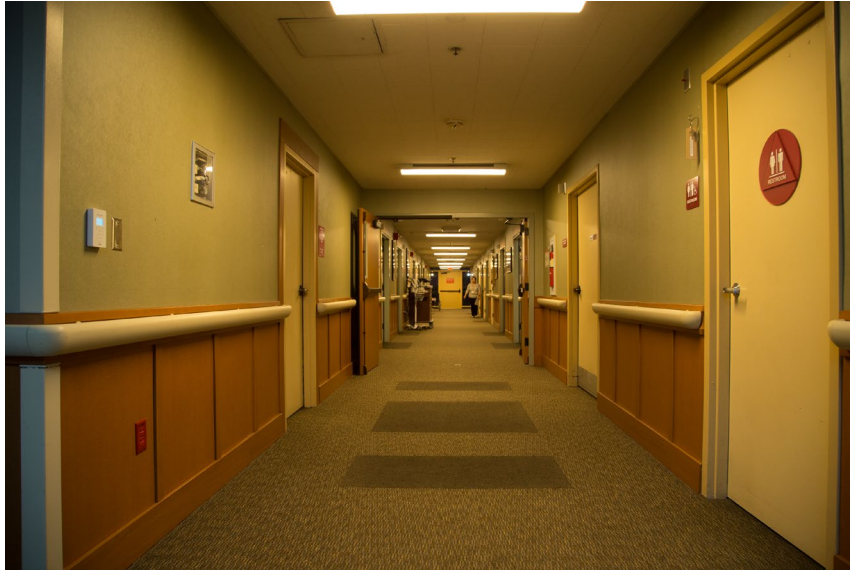
Figure 8. Nighttime corridor lighting, showing 2700 K light setting dimmed to 20% output.
