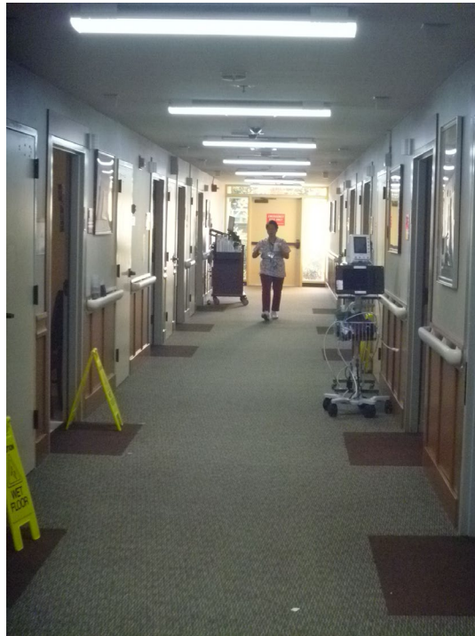
Figure 7. Daytime corridor lighting, showing 6500 K light setting and daylight from windows.
