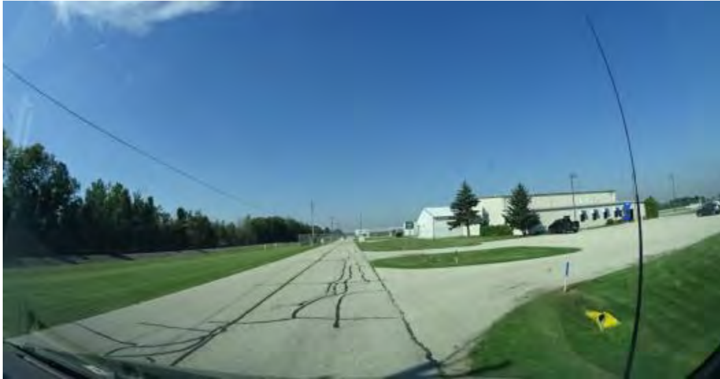
Figure 2-236. Access Road at Potential Rockwood Spur at the Manitowoc Airport Transload Location (Looking North) (2014)
