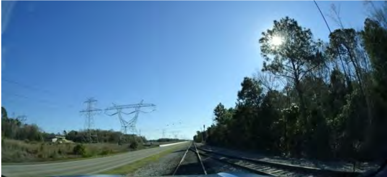
Figure 2-158. Onsite Industrial Rail Spur at the Coal Loop Junction (2015)
