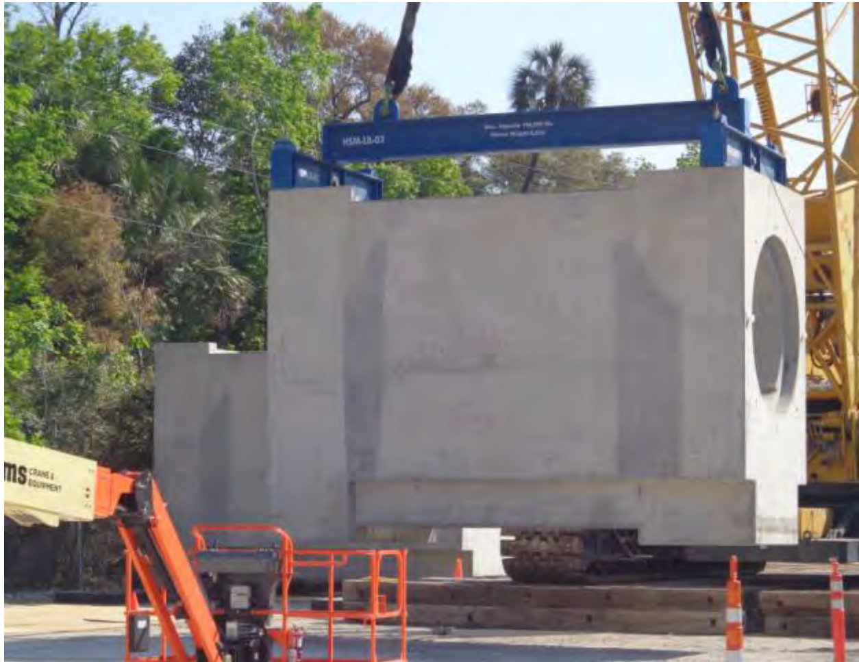
Figure 2-183. Horizontal Storage Module Being Unloaded from Railcar (2015)
