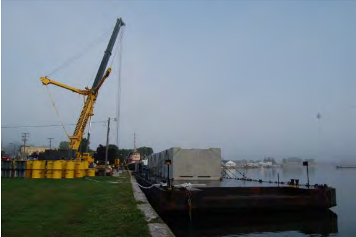
Figure 2-246. Horizontal Storage Modules Being Unloaded from a Barge (2013)
