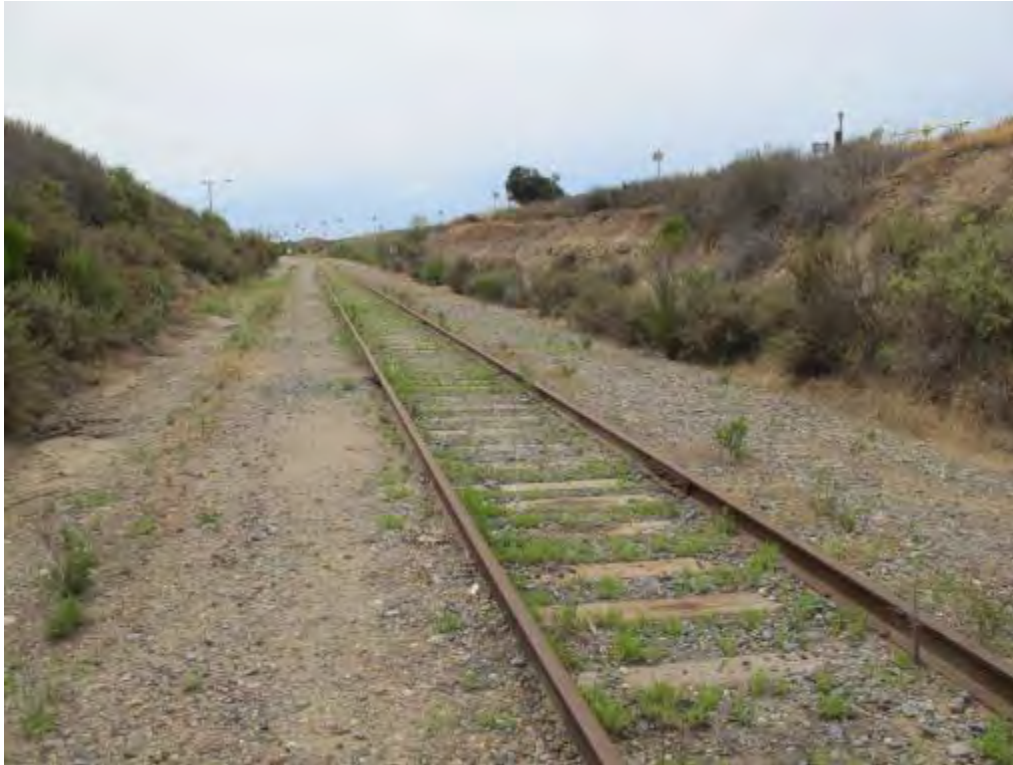
Figure 2-279. Onsite Rail Spur at San Onofre Site (2015)
