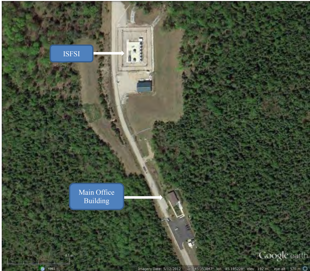
Figure B-3. Closer Satellite View of the Independent Spent Fuel Storage Installation Pad and the Main Office Building at Big Rock Point (Google 2015)
