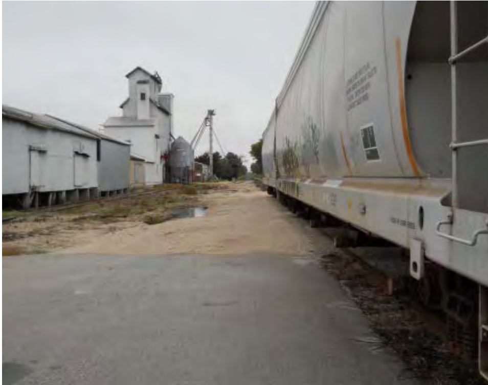
Figure B-41. Siding at Luxemburg (2014)
