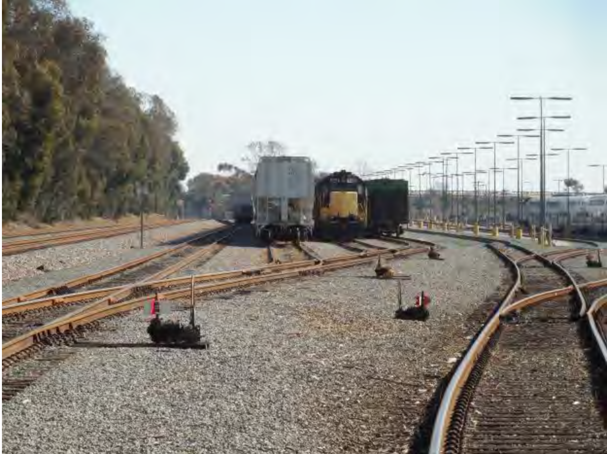
Figure 2-286. Stuart Mesa Rail Yard (Looking South) (2016)
