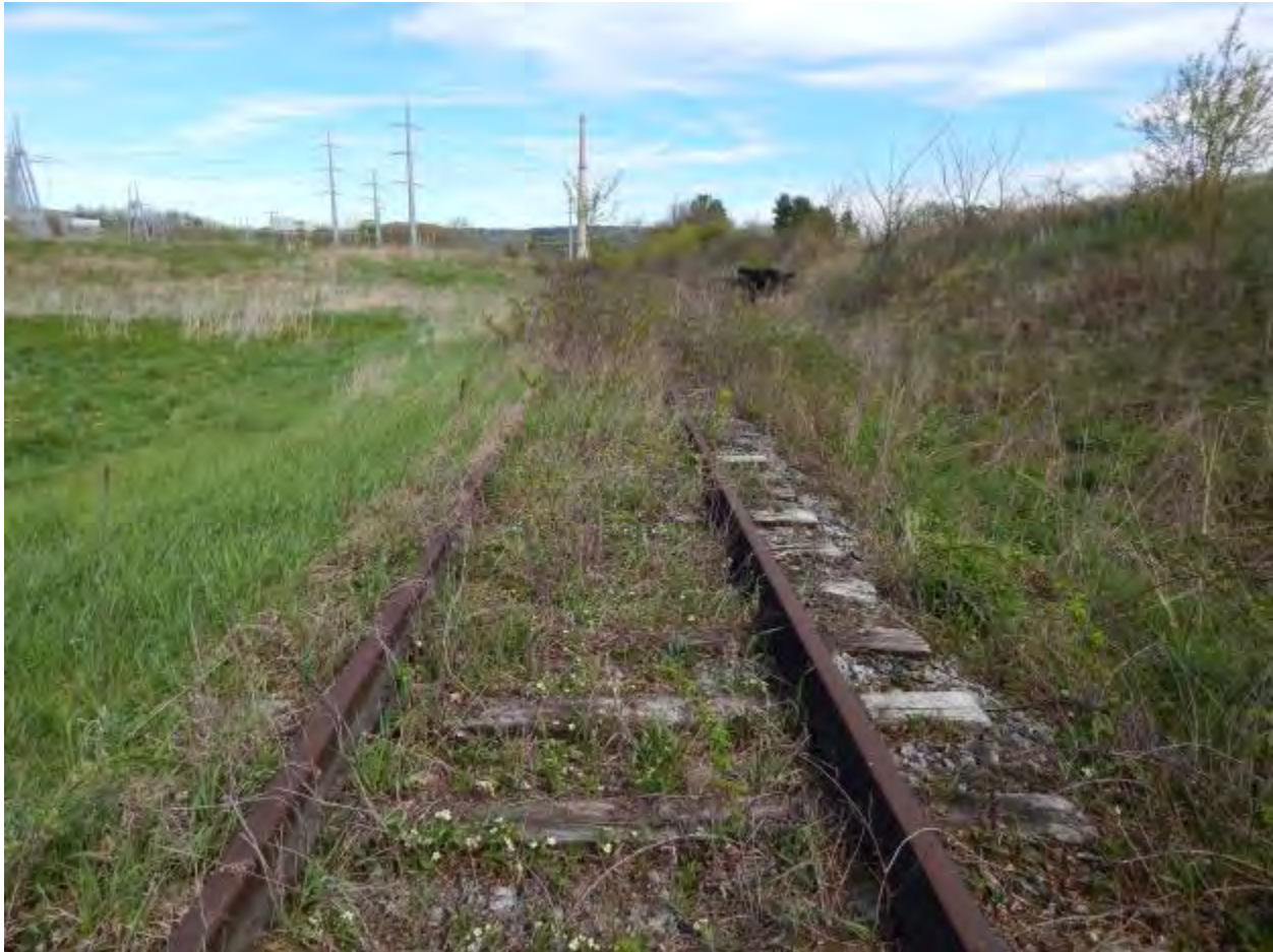
Figure 2-312. Rail Spur Approaching Vermont Yankee Site Entrance (2016)
