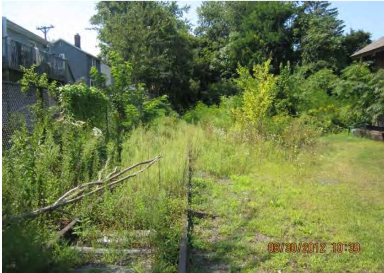
Figure 2-39. Conditions at the End of the Portland Rail Spur (2012)
