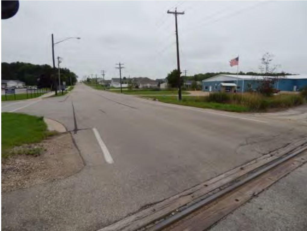
Figure 2-223. Potential Denmark Transload Location (Looking West) (2014)
