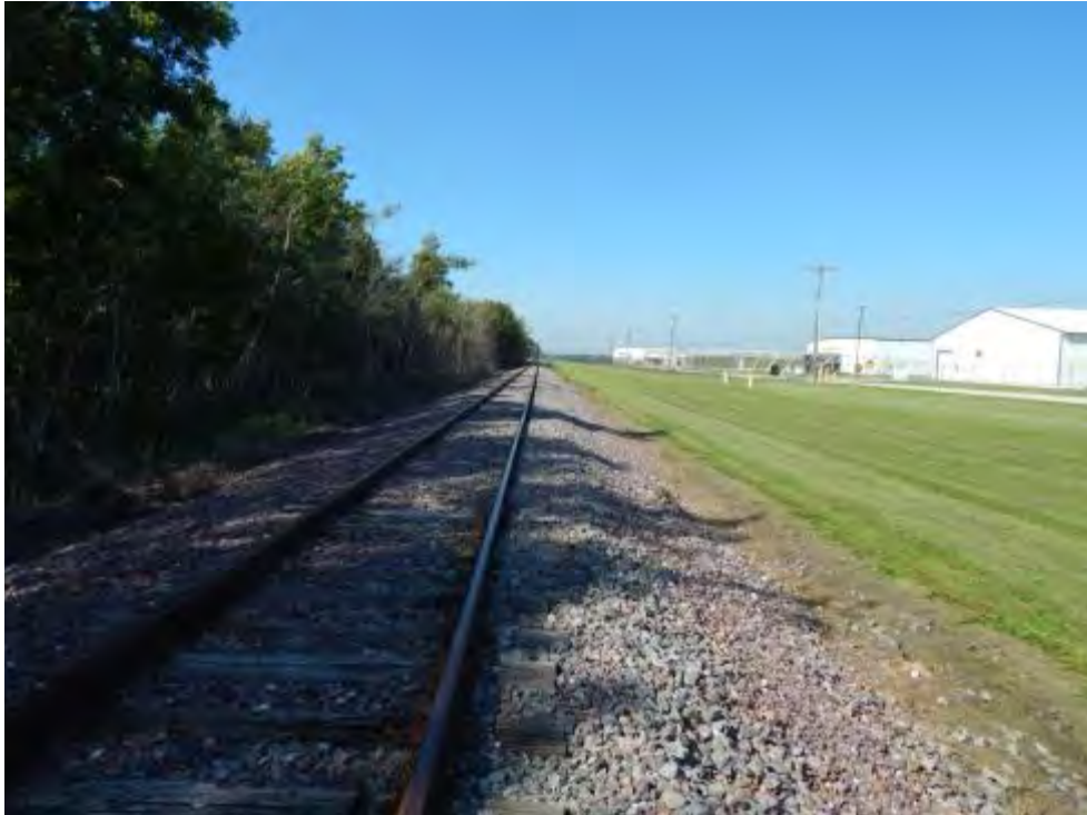
Figure 2-234. Potential Rockwood Spur at the Manitowoc Airport Transload Location (Looking North) (2014)
