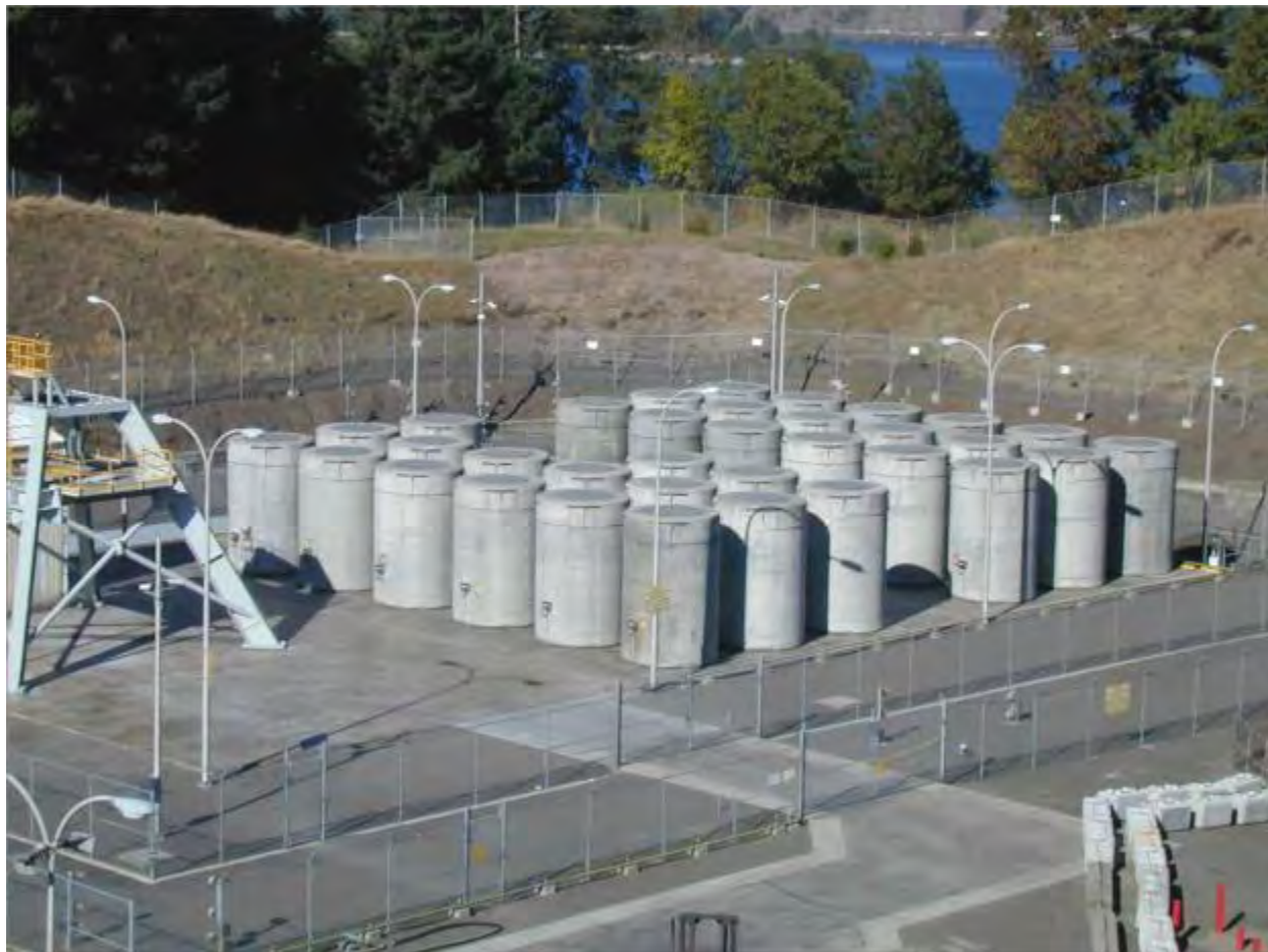
Photo courtesy of Trojan
