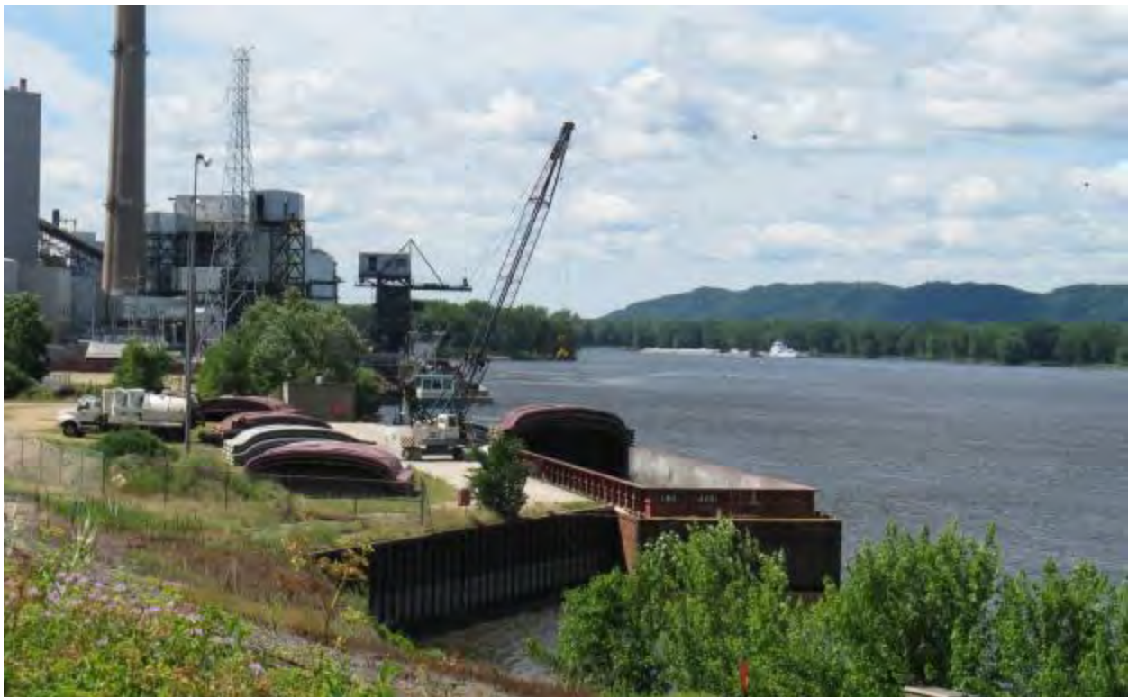
Figure 2-125. Coal Barge at Barge Dock Area at La Crosse Site (2013)
