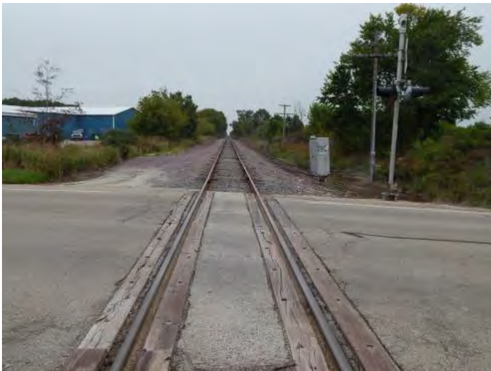
Figure 2-222. Potential Denmark Transload Location (Looking North) (2014)
