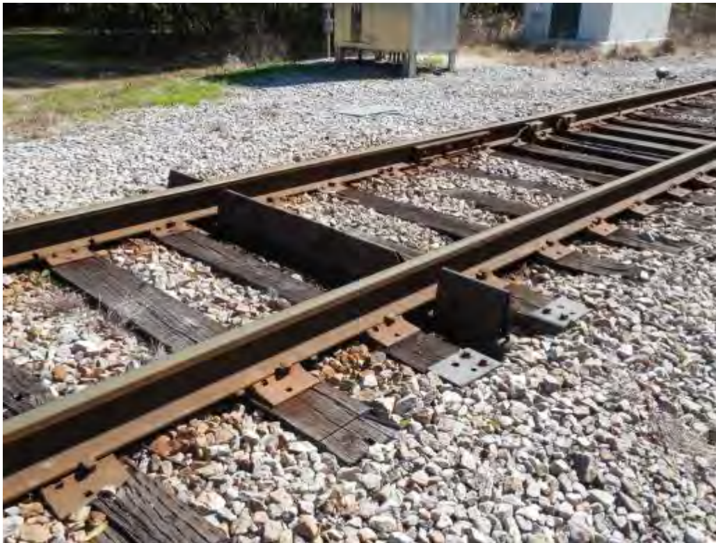
Figure 2-172. Dragging Equipment Detector on Florida Northern Railroad (2015)
