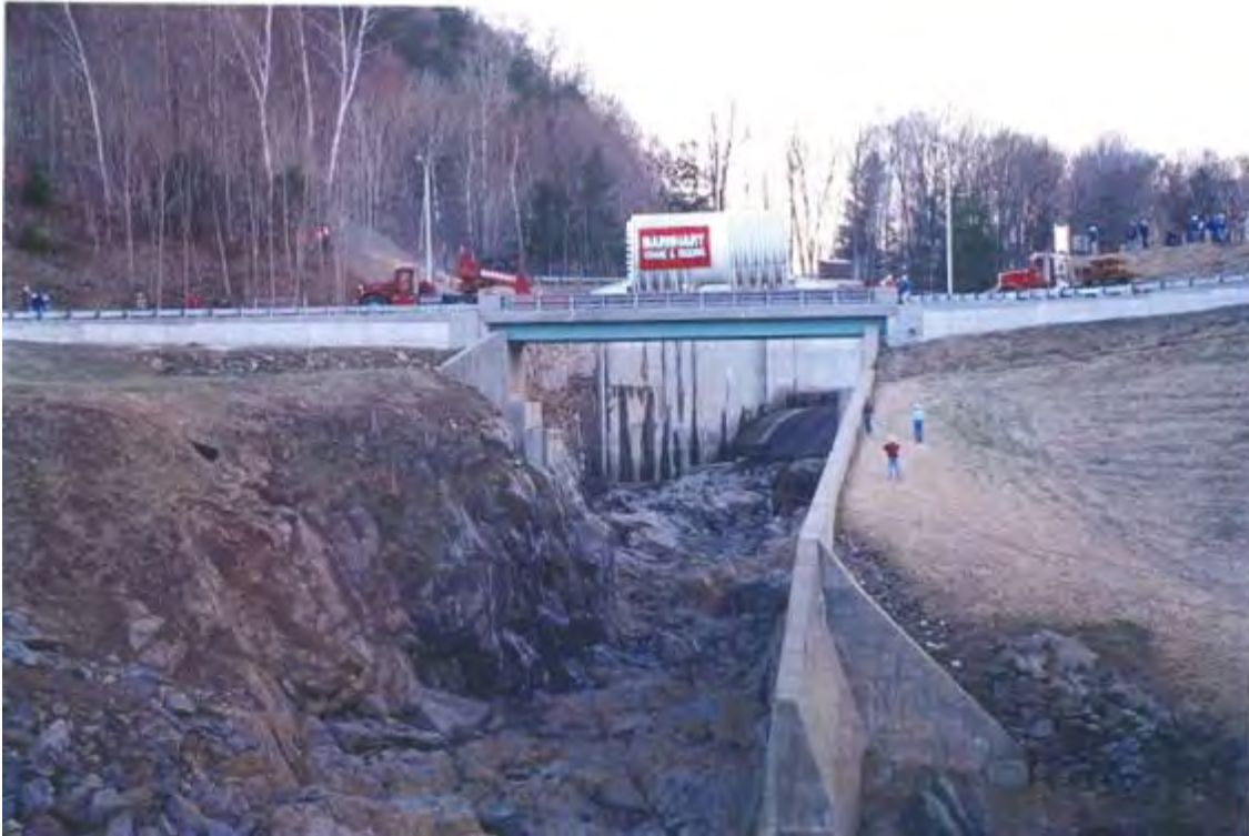
Photo courtesy of AREVA
