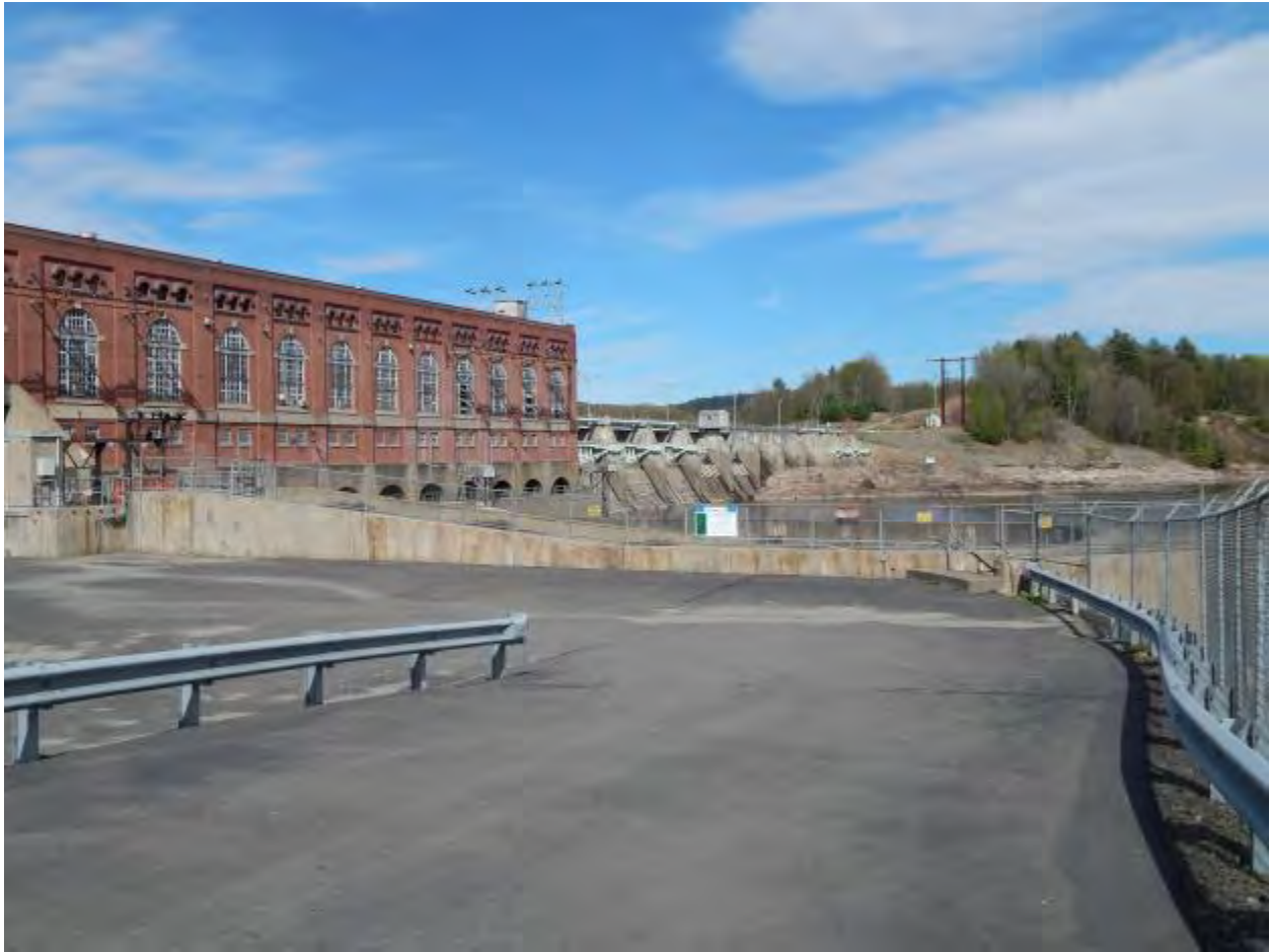
Figure 2-302. Vernon Dam and Hydroelectric Station (2016)
