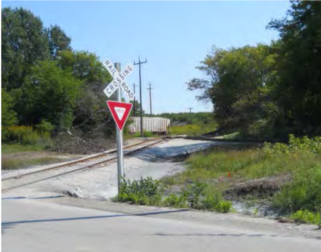
Figure B-32. Switch to Carmeuse Lime Plant and the Country Visions Cooperative Fertilizer Plant Sidings at MP 83.2 (2014)
