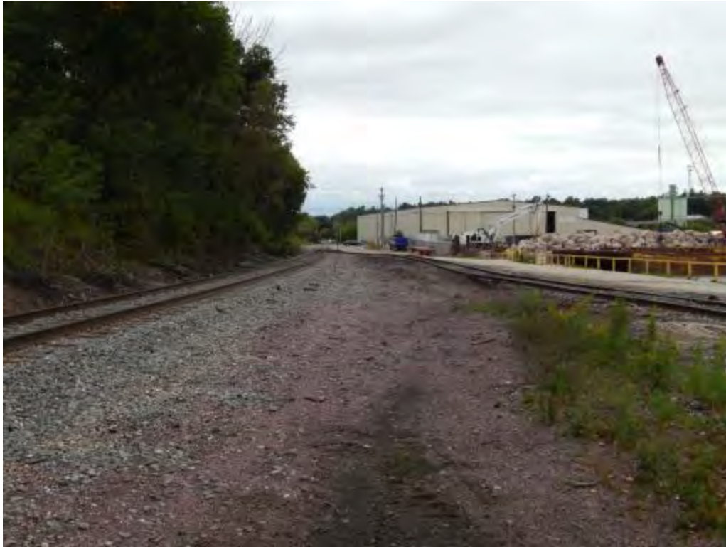
Figure 2-239. Potential Manitowoc Transload Location (Looking Northwest) (2014)
