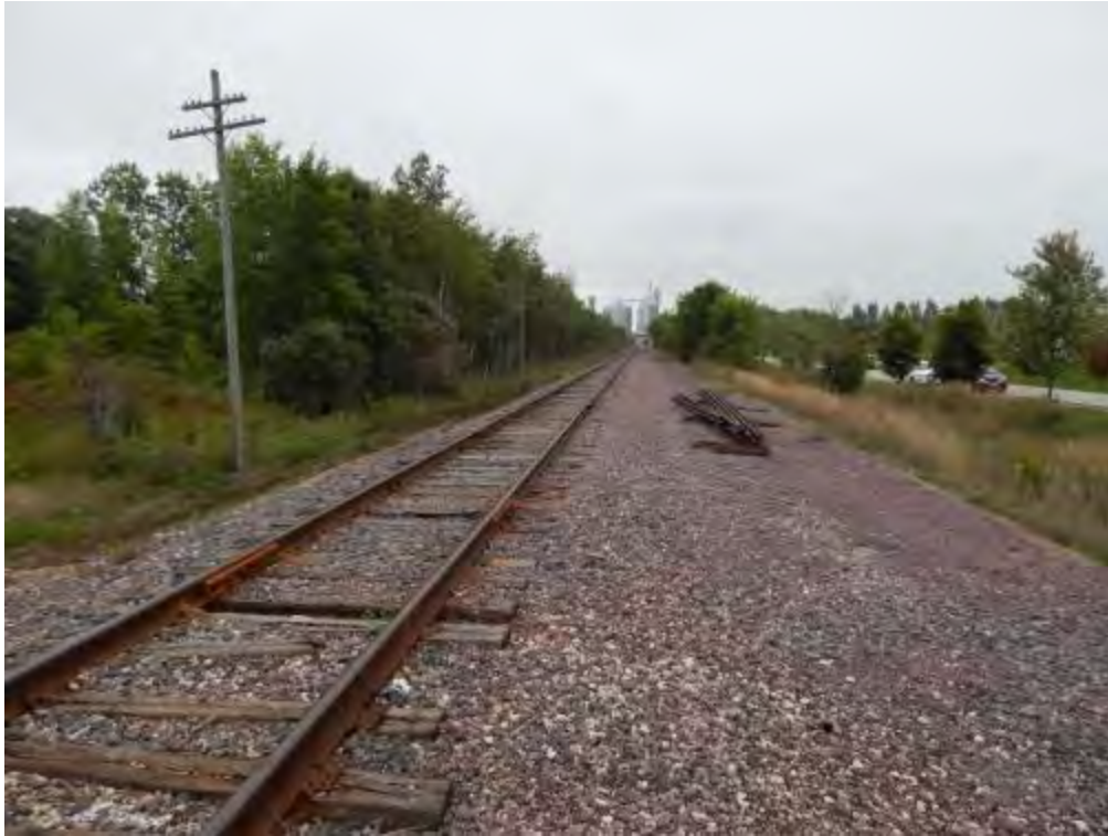
Figure 2-221. Potential Denmark Transload Location (Looking South) (2014)
