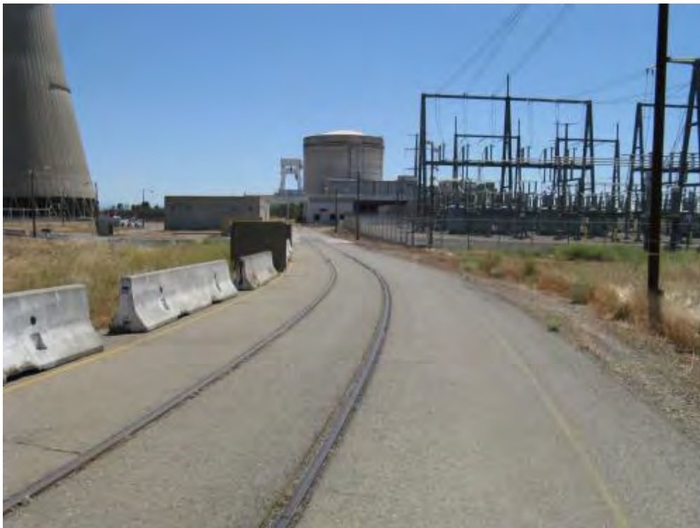
Figure 2-90. On-site Rail Spur Running into Rancho Seco Site (2013)
