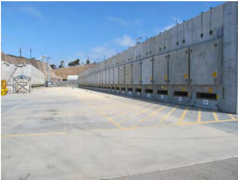
Figure 2-272. Close-up View of San Onofre Independent Spent Fuel Storage Installation (2015)
