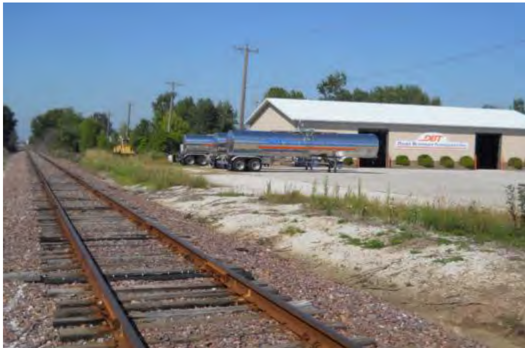
Figure B-35. Dean Brennan Transport Facility (2014)
