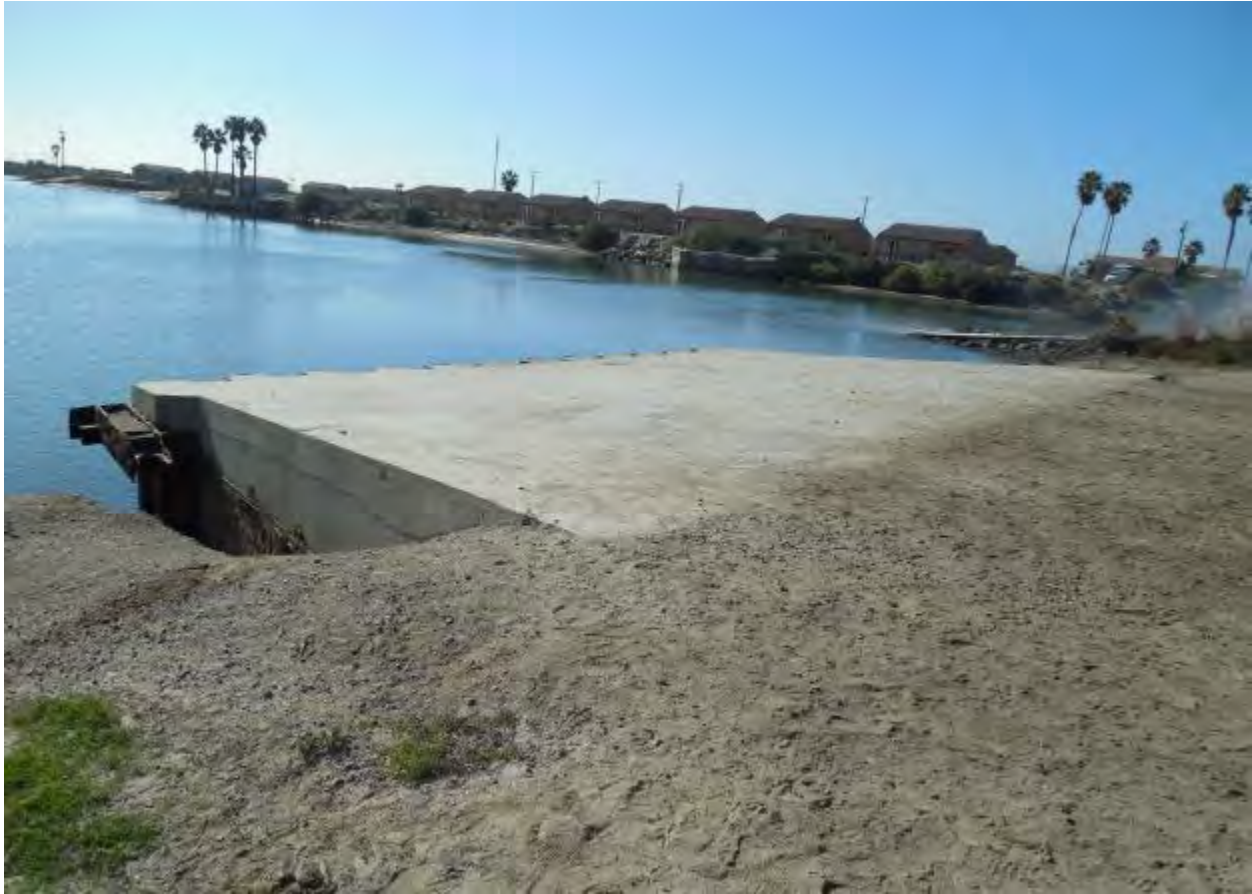
Figure 2-293. Del Mar Boat Basin Bulkhead (2016)
