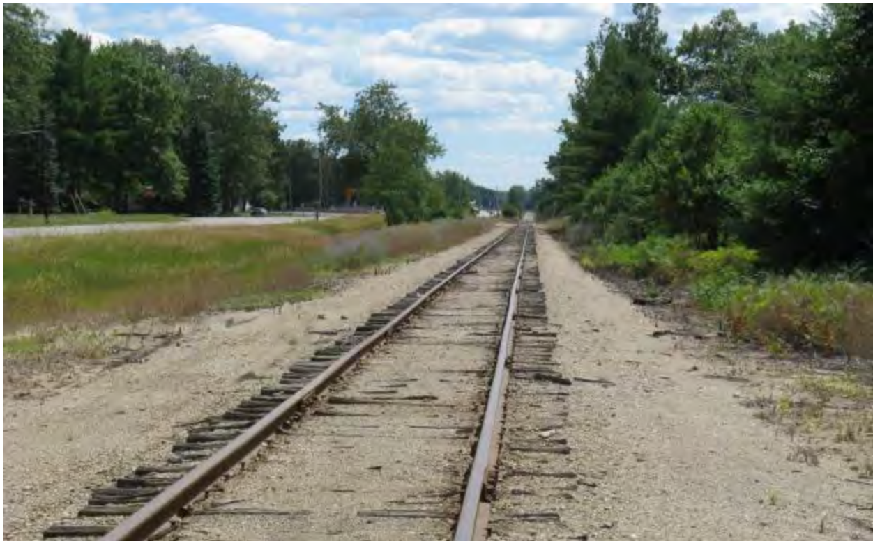
Figure 2-76. Condition of Rail Crossing Used for Big Rock Point Reactor Pressure Vessel Transload (Looking South) (2013)
