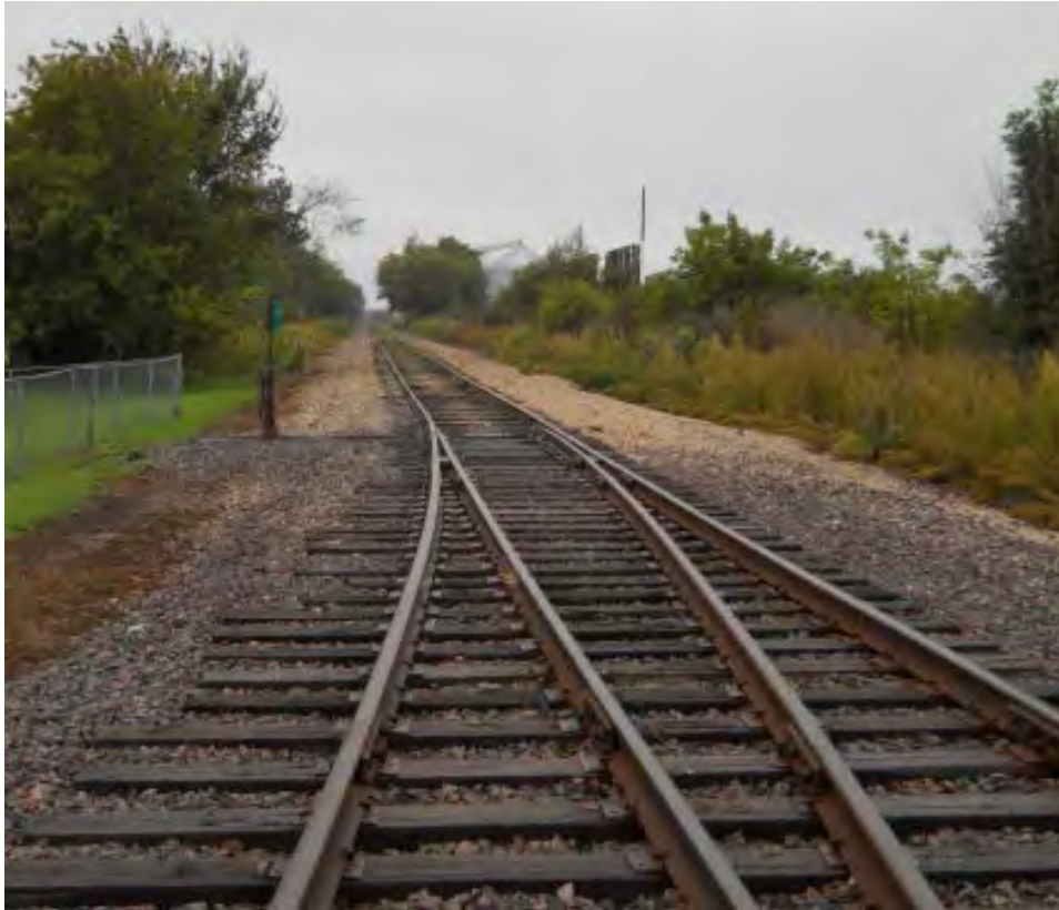
Figure B-43. Switch at Luxemburg (2014)
