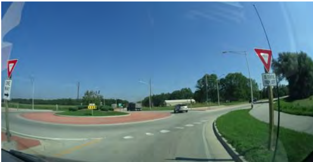
Figure 2-231. Traffic Circle on WI-310 (Looking East) (2014)
