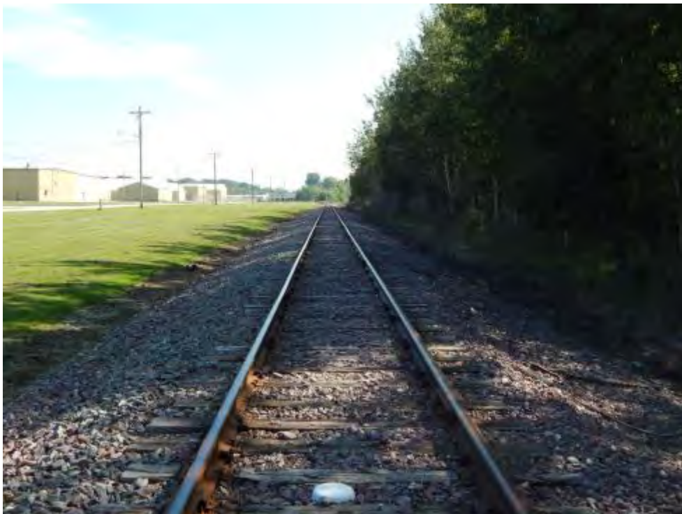
Figure 2-235. Potential Rockwood Spur at the Manitowoc Airport Transload Location (Looking South) (2014)
