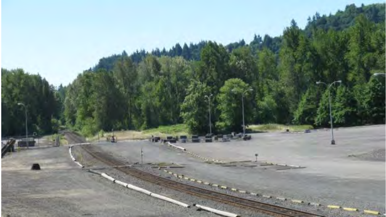
Figure 2-105. Portland and Western Railroad in the Vicinity of the Trojan Site (2013)
