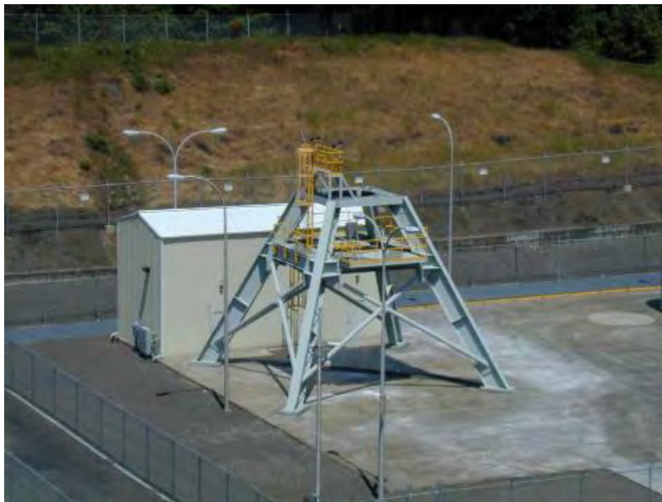
Photo courtesy of Trojan
