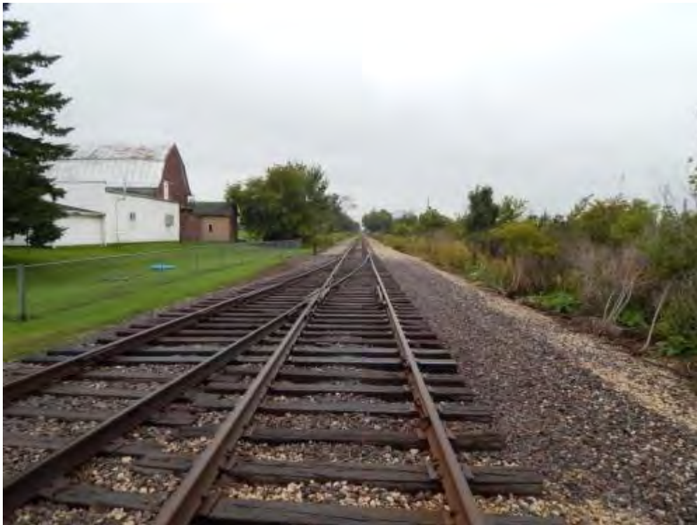
Figure 2-207. Potential Luxemburg Transload Location Further Down Track (Looking West) (2014)
