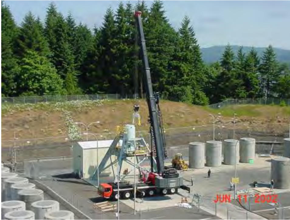
Photo courtesy of Trojan
