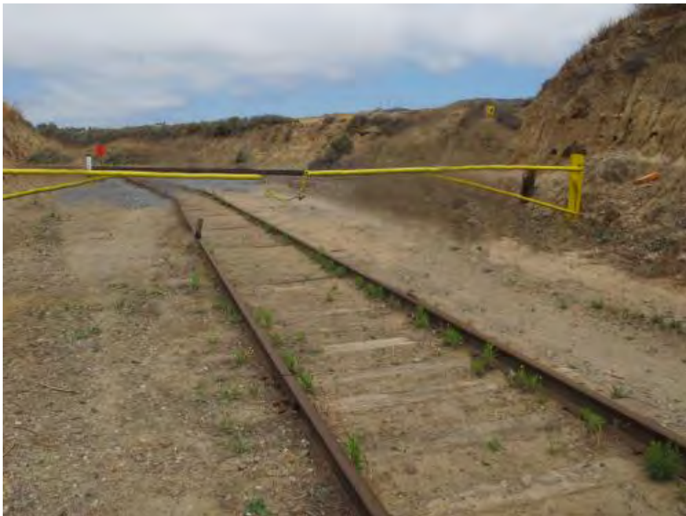
Figure B-58. Locked Facility Gate (2015)
