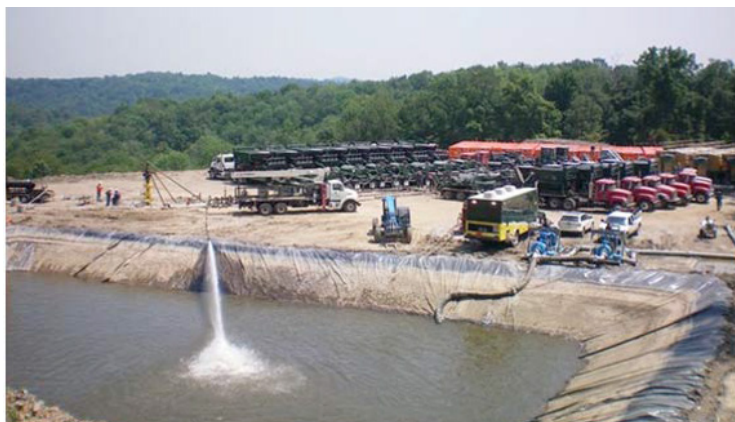
Lined impoundments provide temporary storage of water needed for hydraulic fracturing. (NETL's E&P Focus Newsletter )
