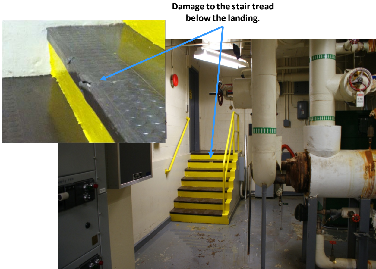
Figure 5: Damaged Edge of the Second Step on Mechanical Equipment Room 7 Stairs
