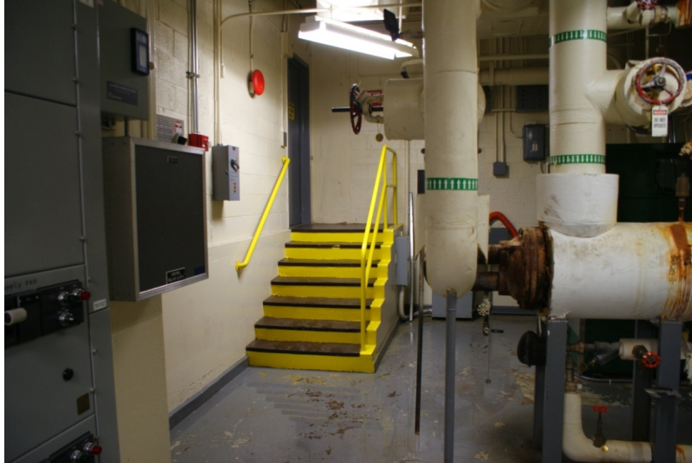
Figure 3: Mechanical Equipment Room 7 Entrance Stairs
