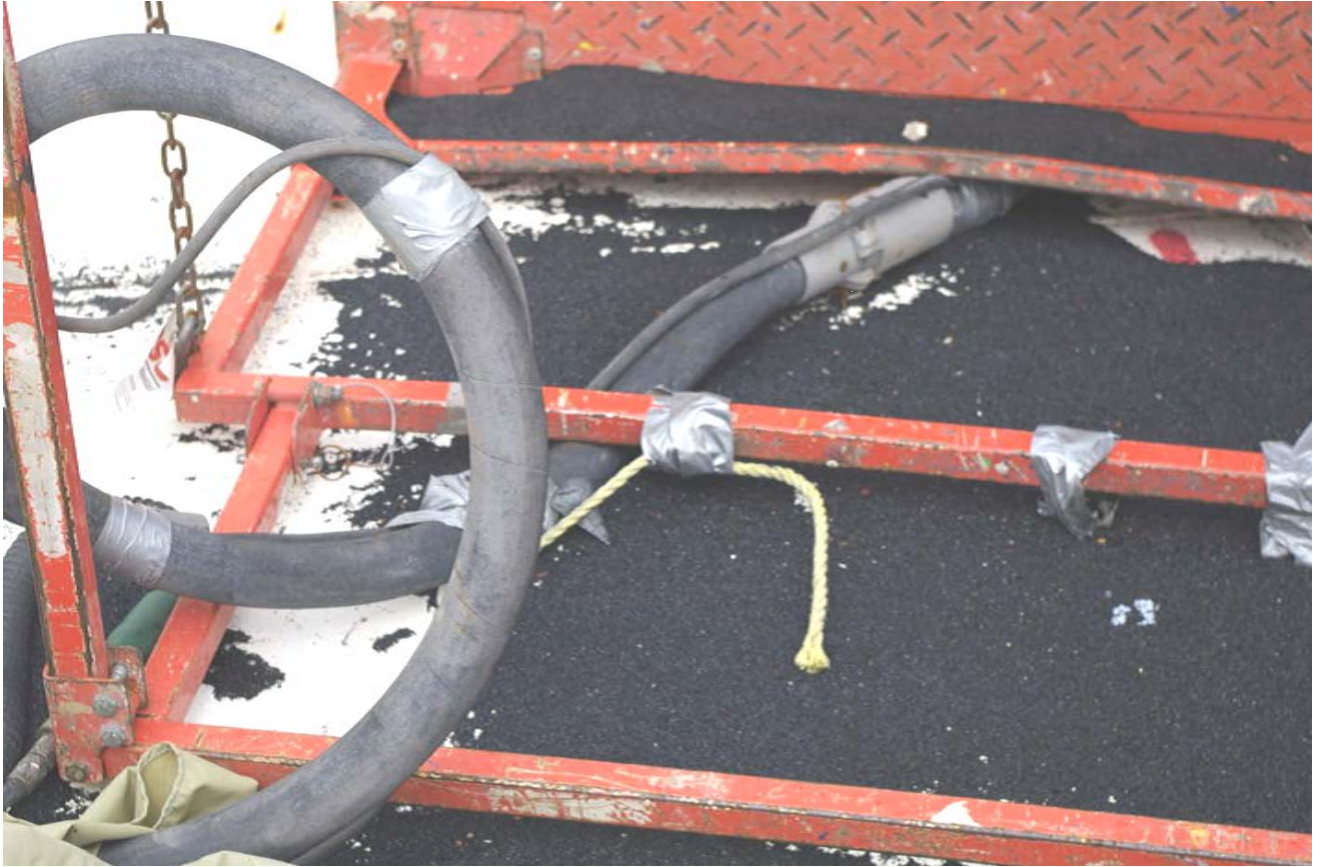
Figure E-8: Platform of Scissor Lift with Blasting and Electrical Control Cable Attached
