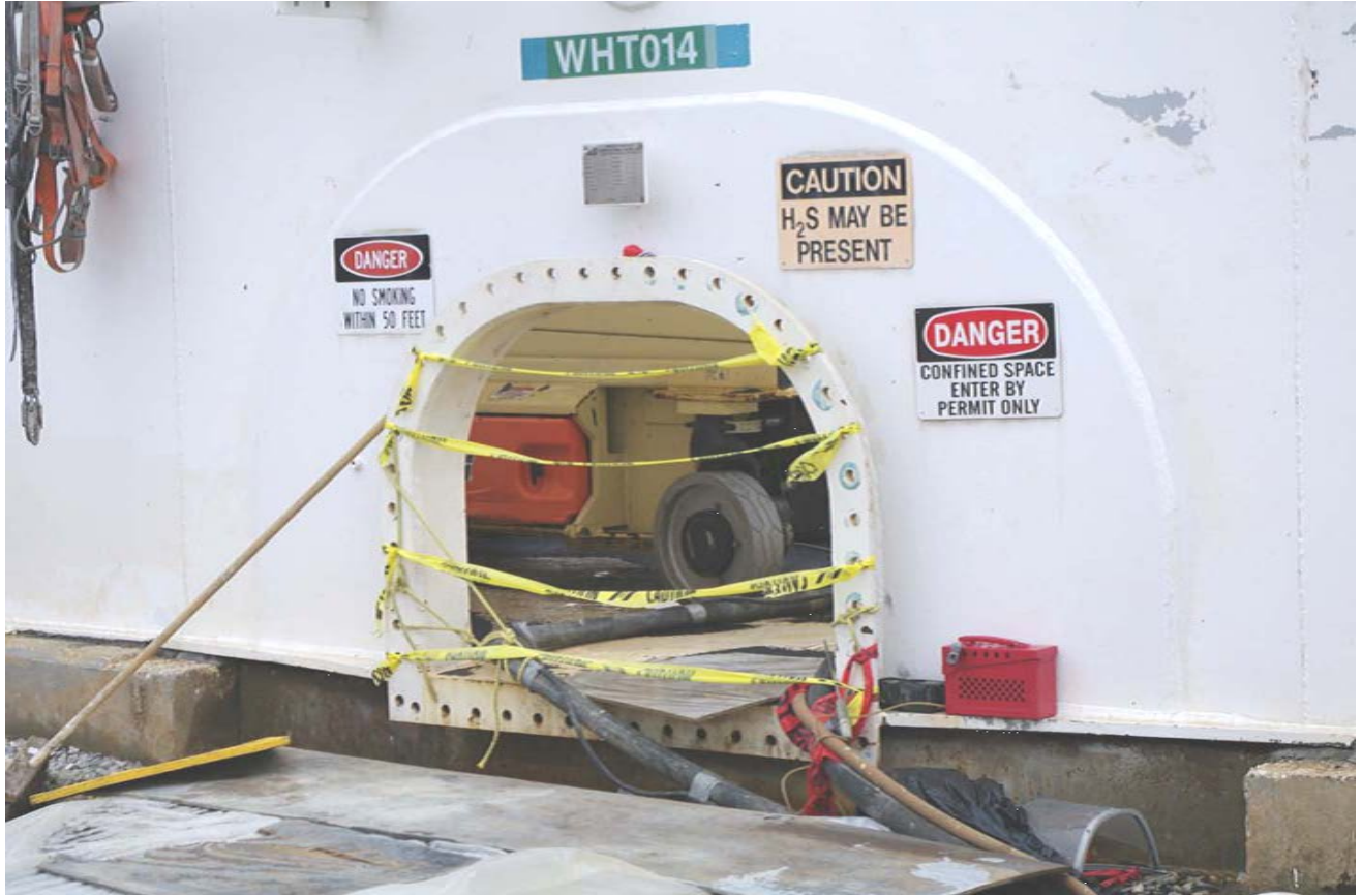
Figure E-5: Outside Manhole of WHT-14
