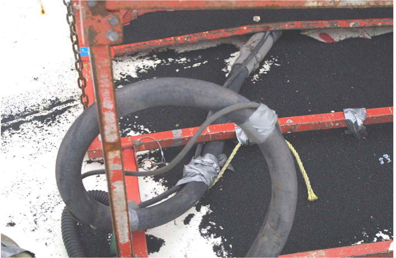
Figure E-9: Close-up of Blasting and Electrical Control Cable Attached to Work Platform Guardrails
