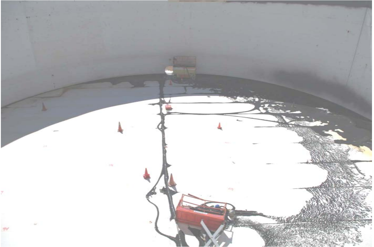
Figure E-2: WHT-14 and Scissor Lift in Relation to Manhole
