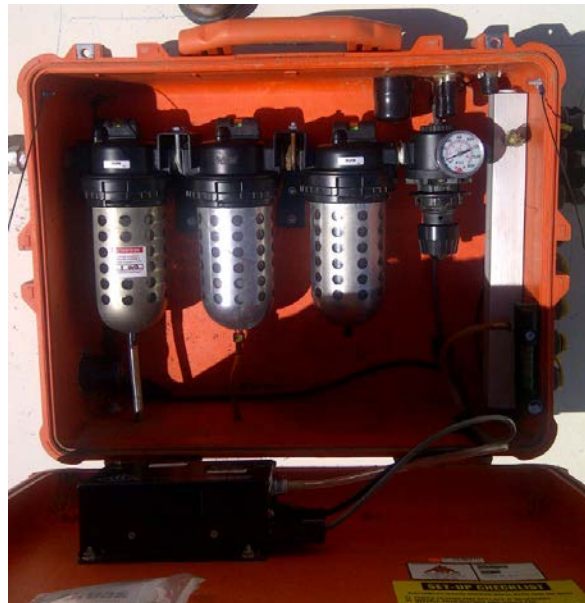
Figure 9: Breathing Air Filtration System
