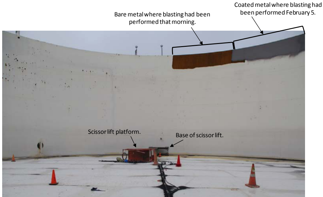
Figure 11: Position of the scissor lift in relation to work completed.
