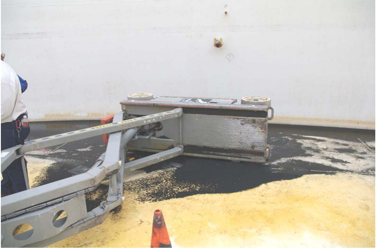
Figure E-4: Base of Scissor Lift in WHT-14
