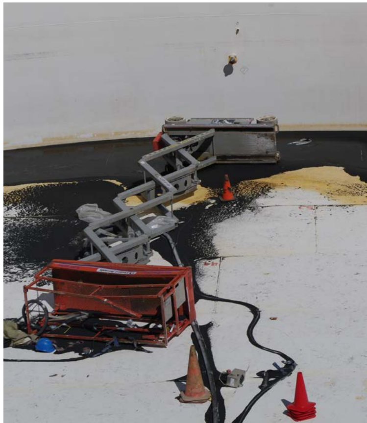
Figure 6: Overturned Scissor Lift in Tank
