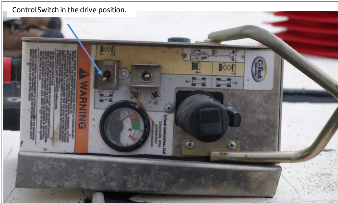
Figure 12: Control Box with three-way switch pointing to the drive position
