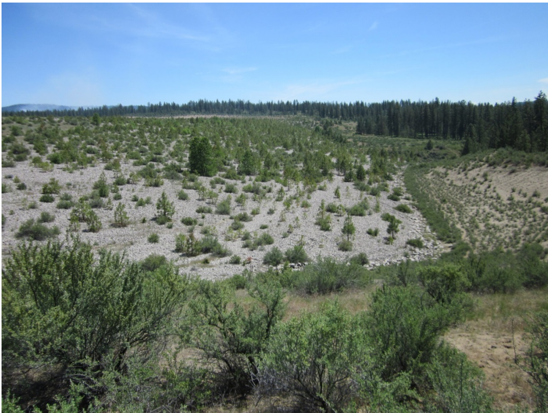
SHE 4/2015. PL-6. 5/2015. Face of tailings dam, view to east.
