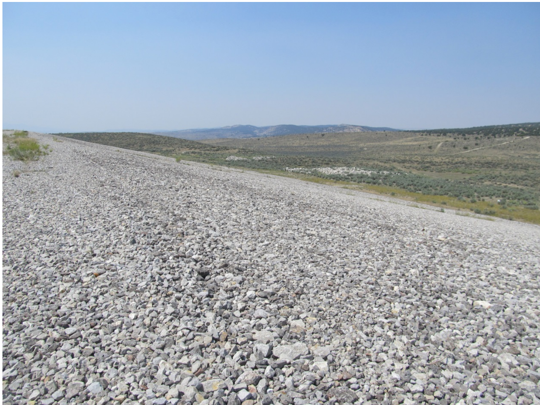
MAW 8/2015. PL-7. Northeast side slope of the disposal cell.
