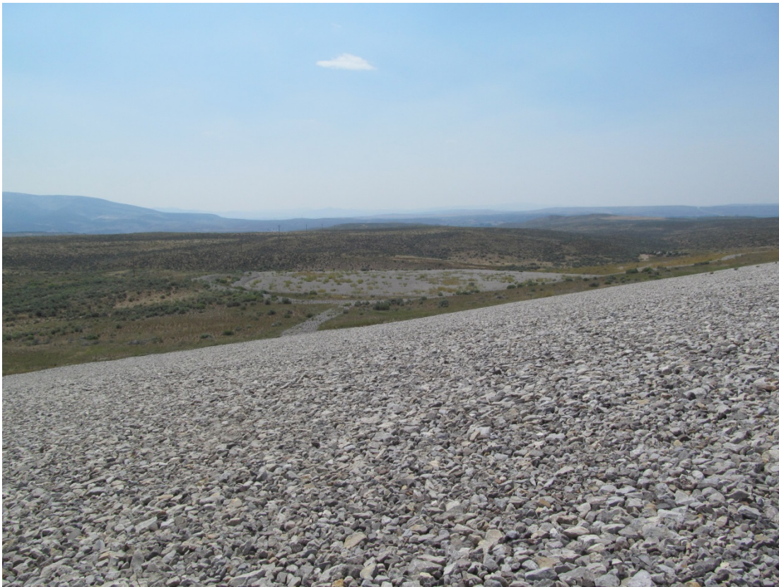
MAW 8/2015. PL-8. South side slope of the disposal cell; ancillary cell in the background.
