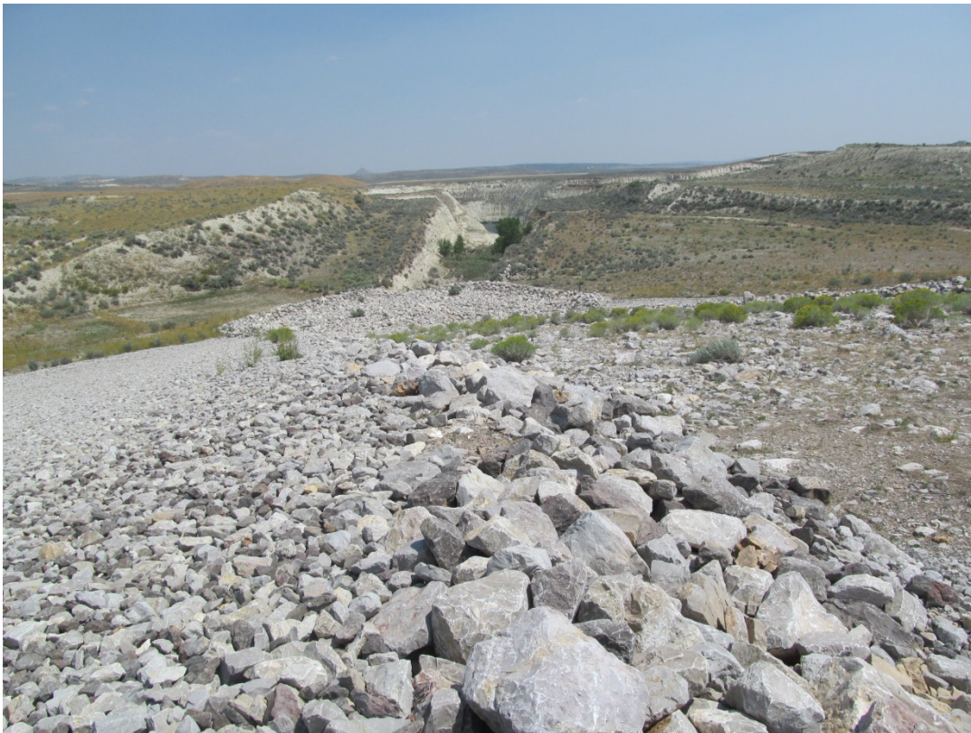
MAW 8/2015. PL-10. Diversion Channel No. 1 outlet into the launch rock erosion protection basin on the east side slope of the disposal cell; Rob Pit in background.
