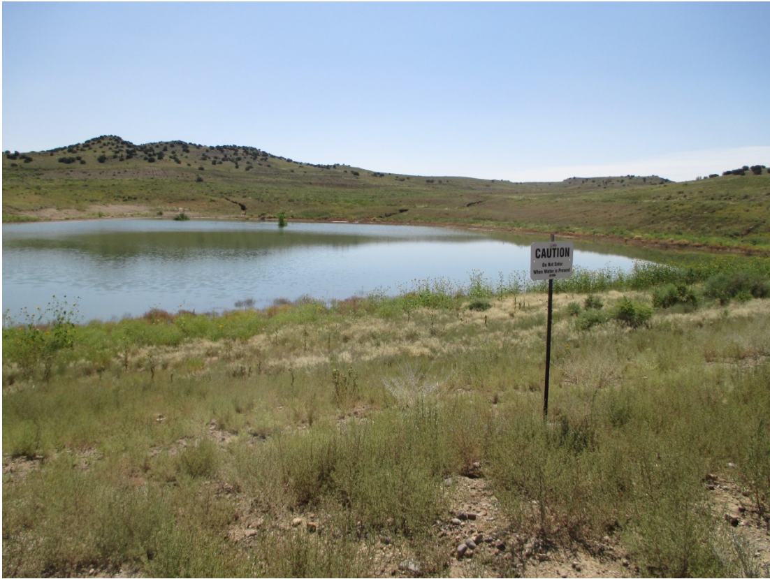
BAR 8/2015. PL-8. Ponded water in sediment trap.
