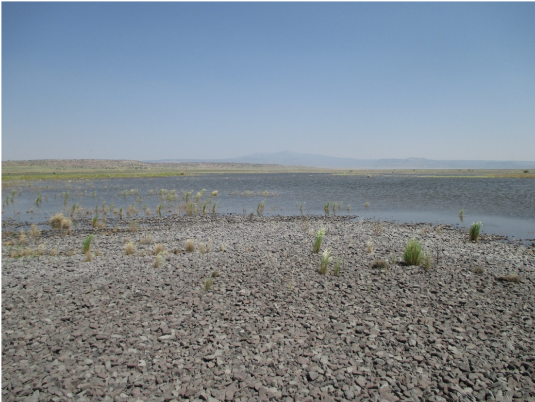
BLU 8/2015. PL-8. Ponded water on north end of main tailings disposal cell top slope.
