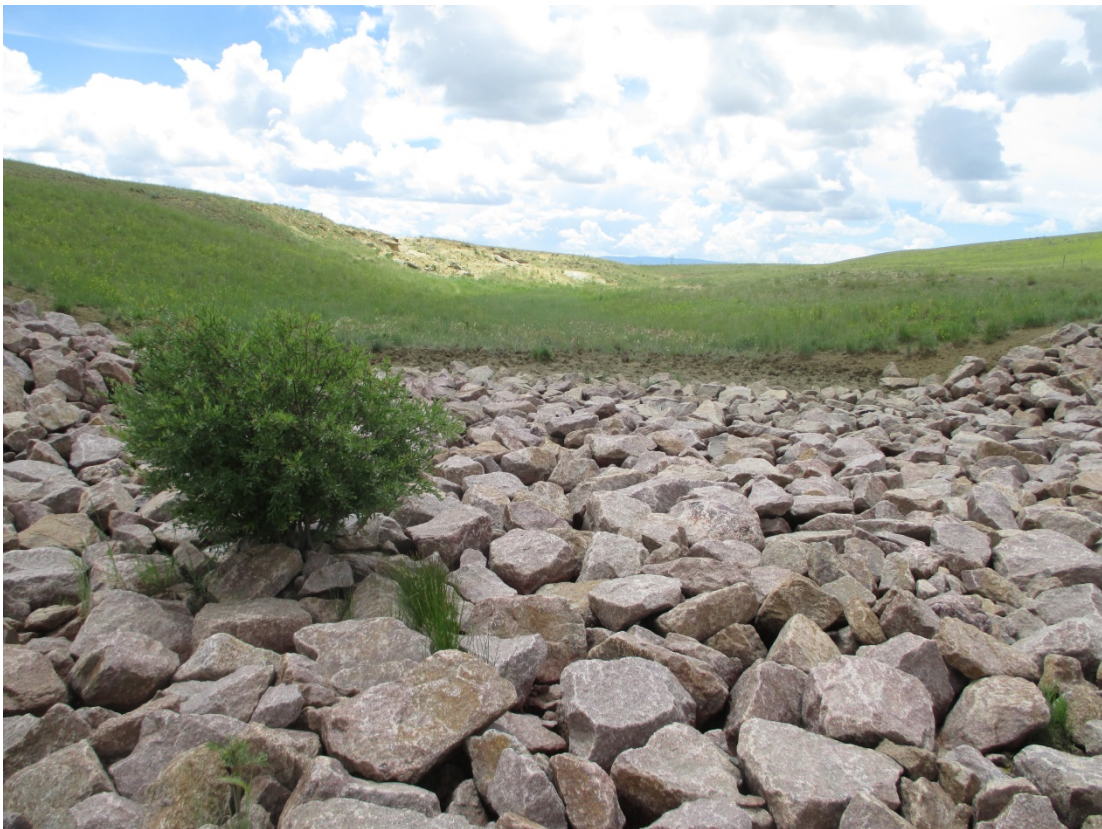
SBS 7/2015. PL-8. Outlet of rock-armored north channel.
