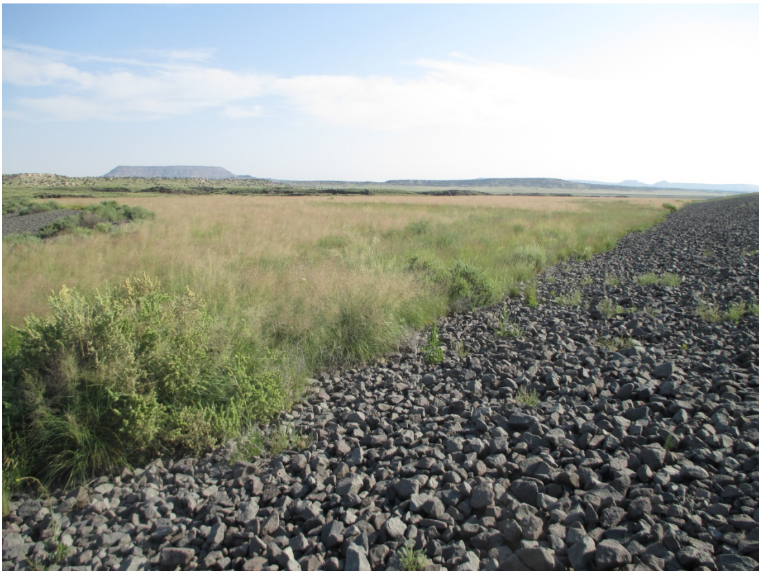
BLU 8/2015. PL-4. Acid tailings bench of main tailings disposal cell.
