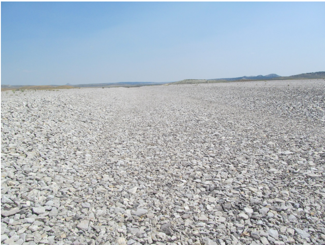
MAW 8/2015. PL-9. Diversion Channel No. 1; view downslope.
