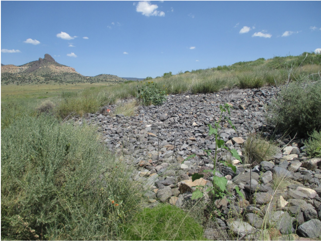
BAR 8/2015. PL-6. Rock-armored slope of containment dam.
