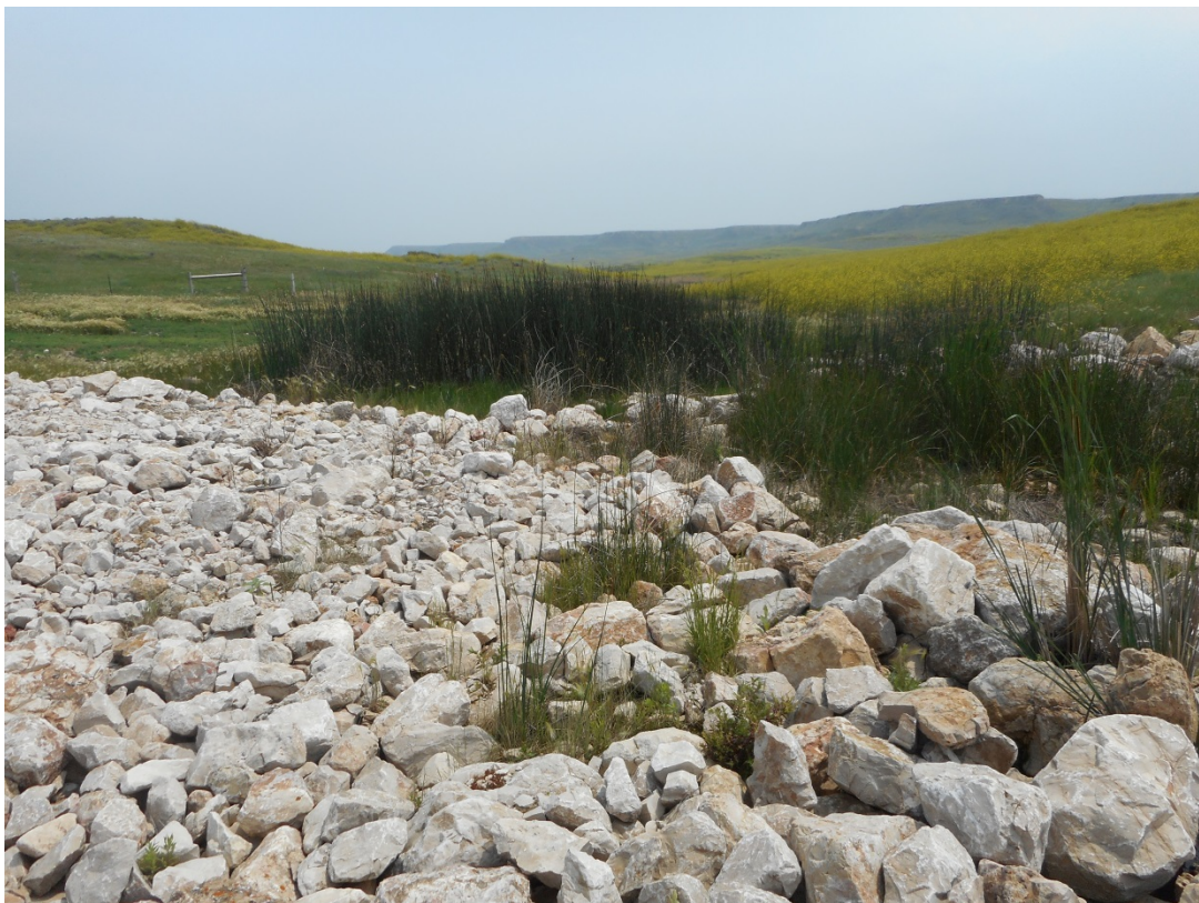
EDG 7/2015. PL-6. Wetland vegetation at base of embankment.
