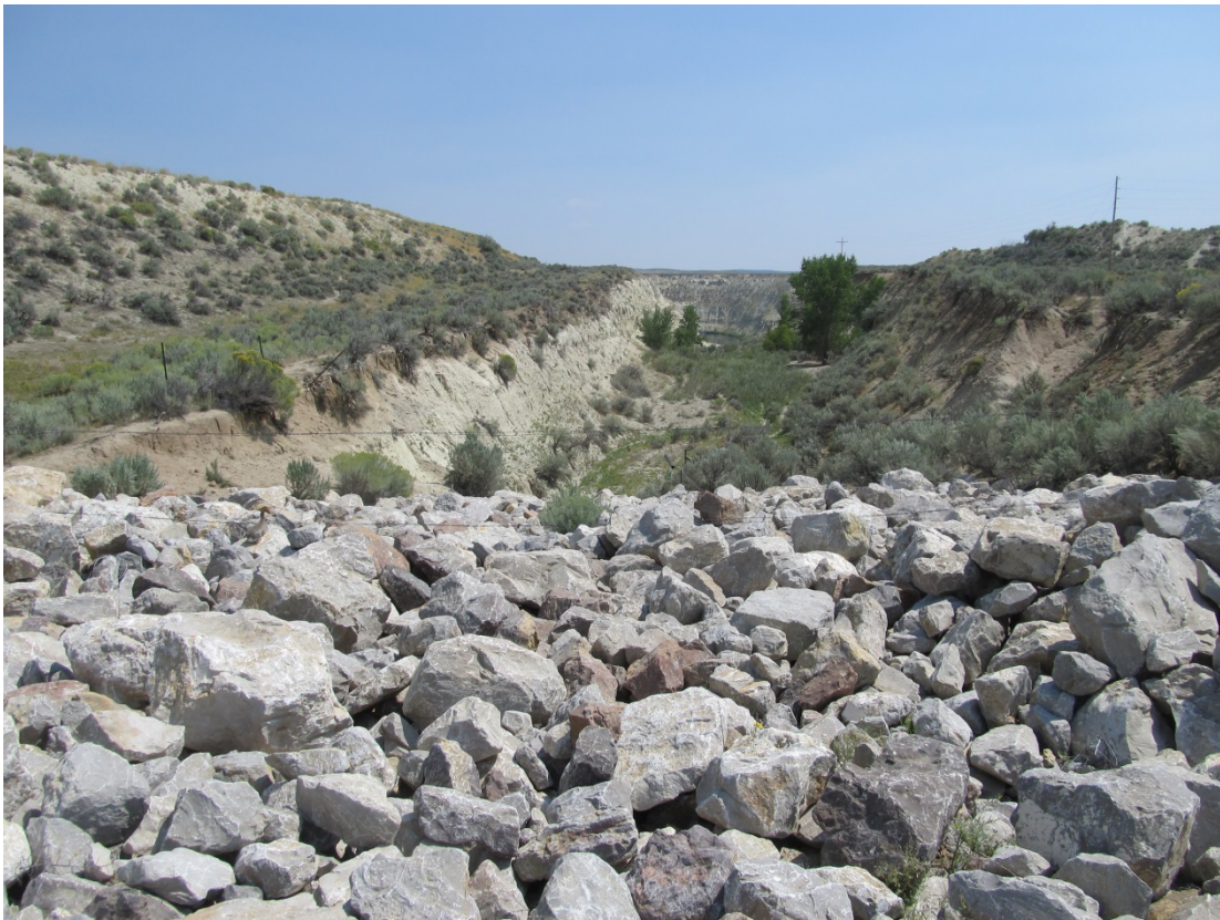
MAW 8/2015. PL-12. Diversion Channel No. 1 outlet channel; Rob Pit in background.
