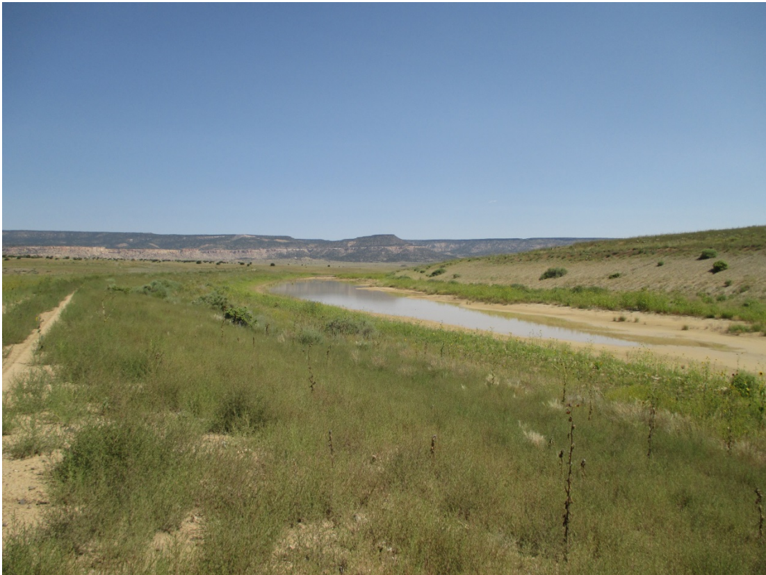
BAR 8/2015. PL-7. Ponded water in east diversion channel.
