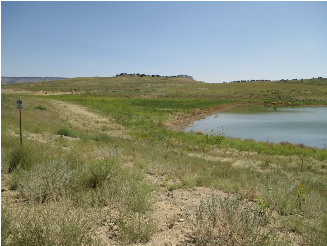
BAR 8/2015. PL-9. Area where ponded water in sediment trap spilled into east diversion channel.
