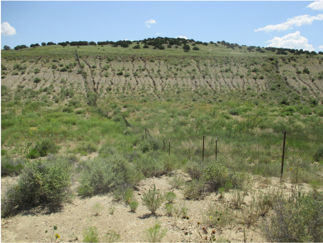
BAR 8/2015. PL-10. Slope erosion and sediment deposition in the south diversion channel.
