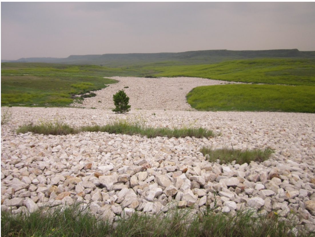
EDG 7/2015. PL-4. Tailings embankment, looking southeast.
