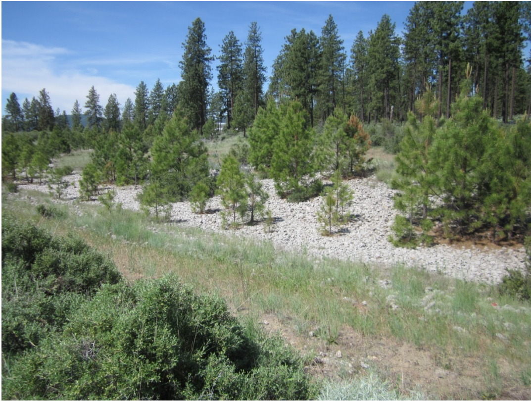
SHE 4/2015. PL-5. 5/2015. Diversion channel, west side of dike road.
