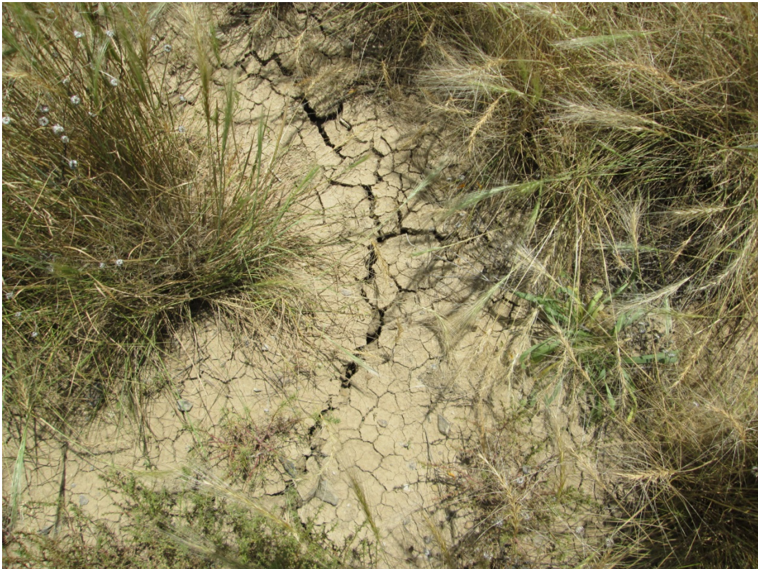
BAR 8/2015. PL-5. Desiccation cracks on the tailings impoundment top slope.
