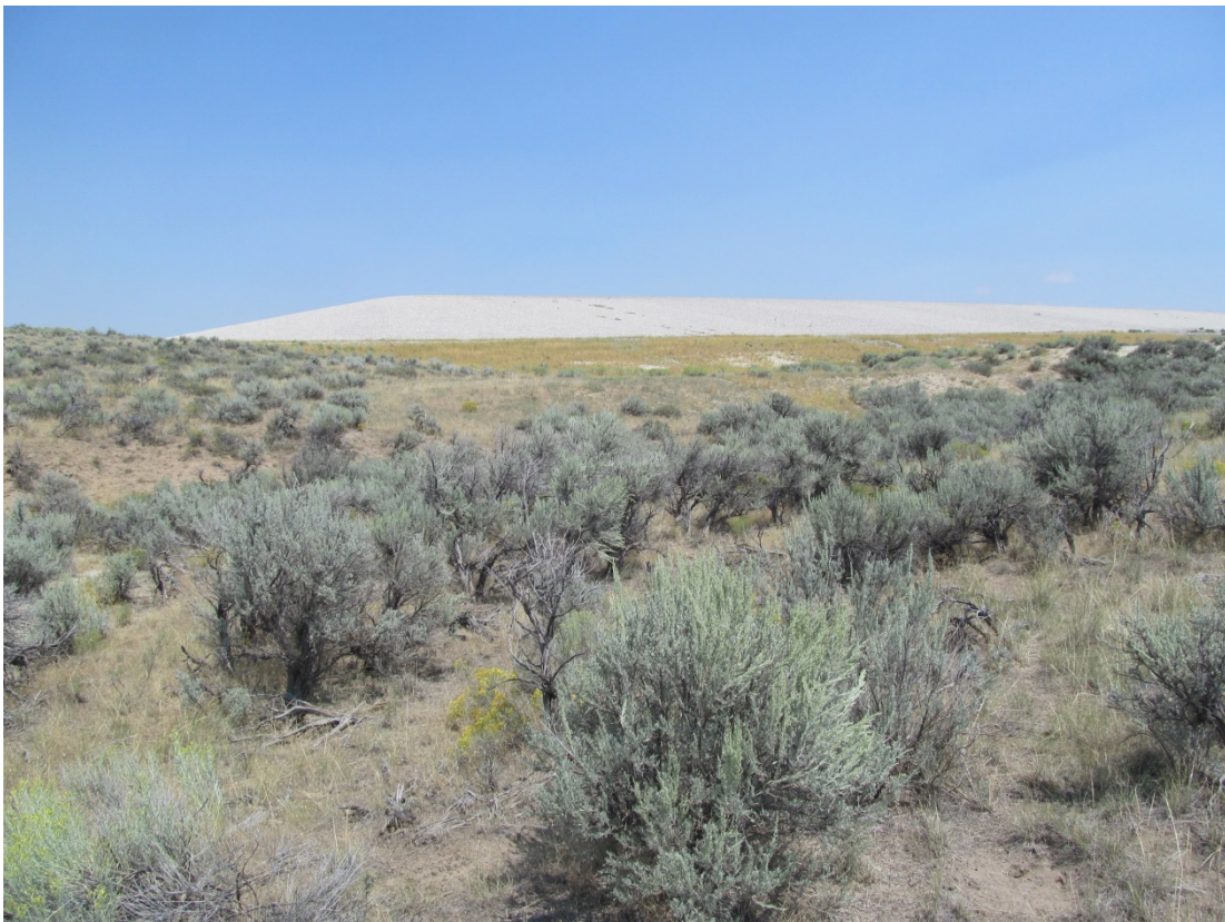
MAW 8/2015. PL-5. Southwestern portion of the site; disposal cell in background.
