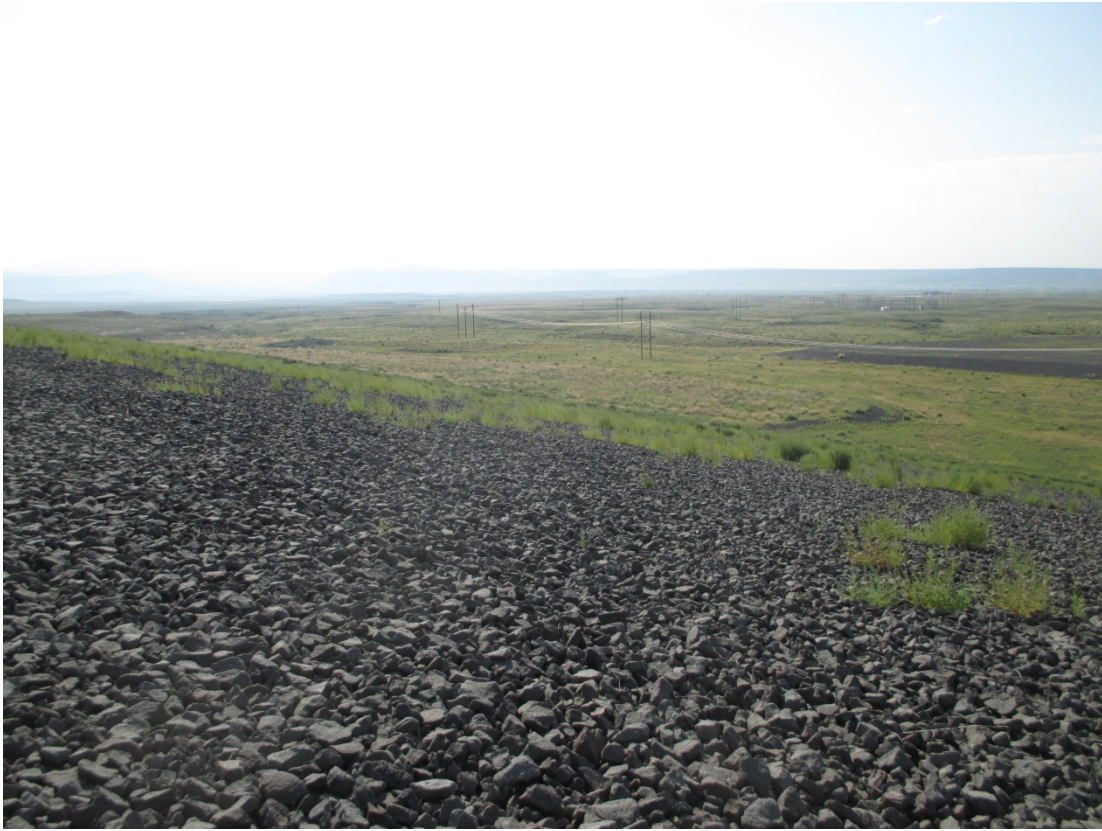
BLU 8/2015. PL-5. South bench of main tailings disposal cell.
