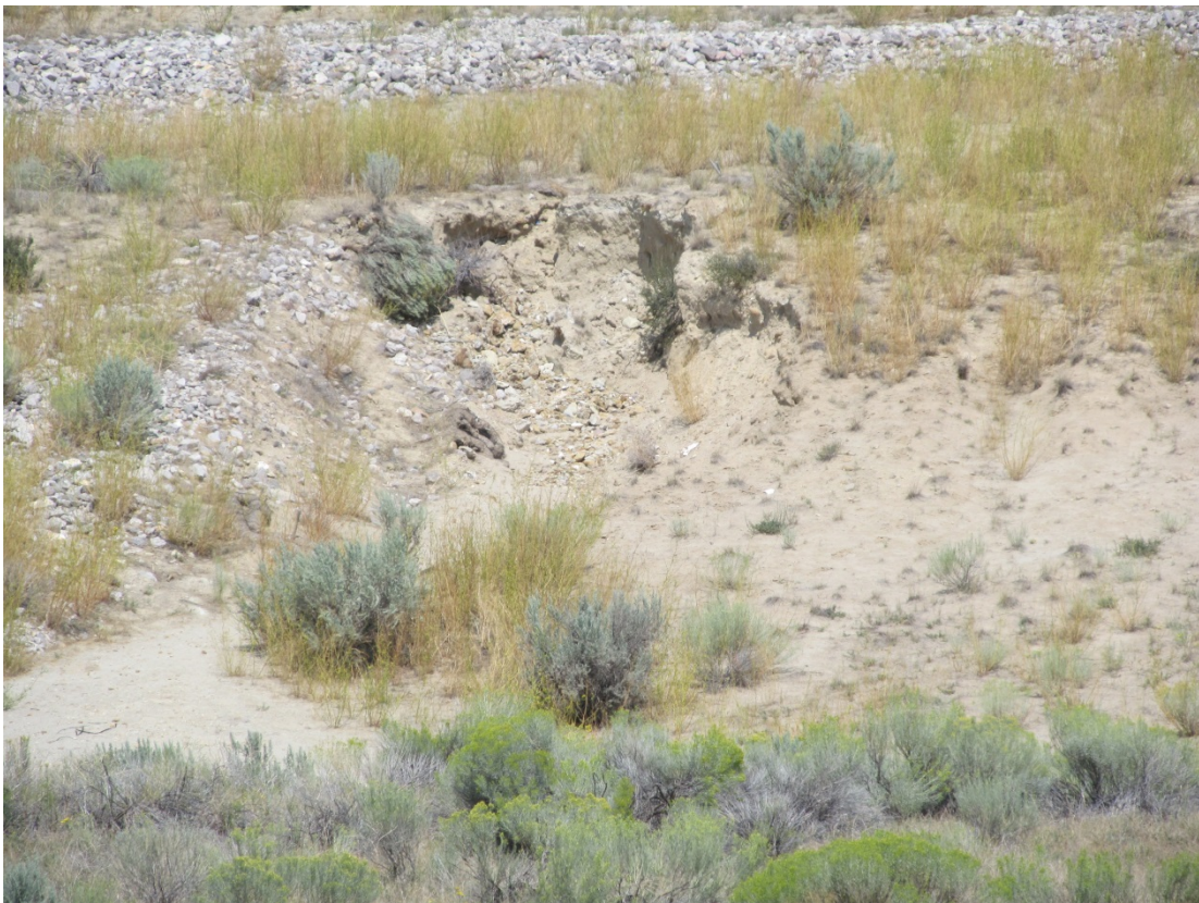
MAW 8/2015. PL-13. Gully on slope south of disposal cell.
