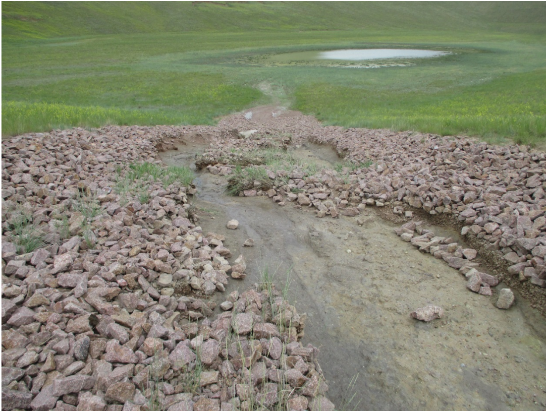
SBS 7/2015. PL-11. Eroded rock-armored channel in south end of Pit 4.
