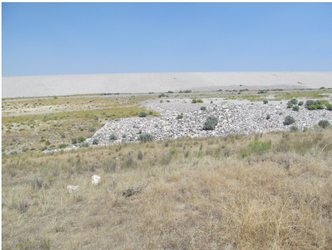
MAW 8/2015. PL-11. Diversion Channel No. 2 outlet and ancillary cell; main disposal cell in background.
