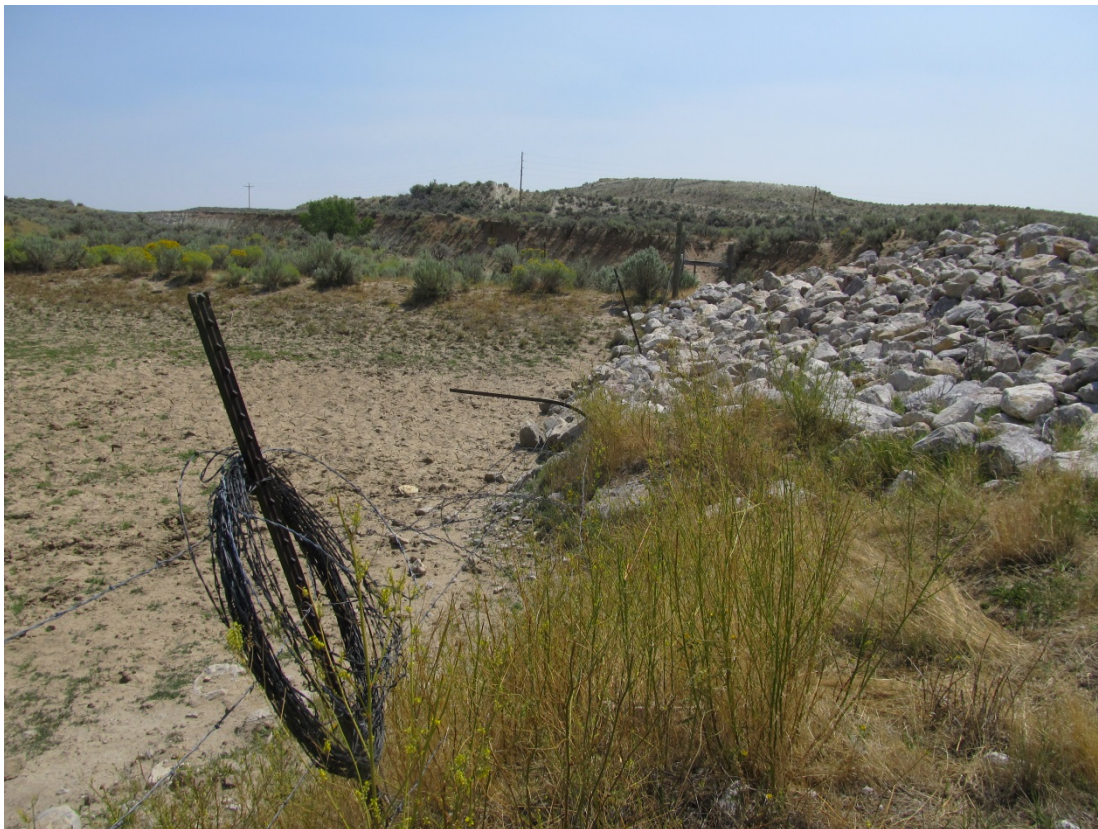
MAW 8/2015. PL-1. Fence damage near Diversion Channel No. 1 outlet channel.
