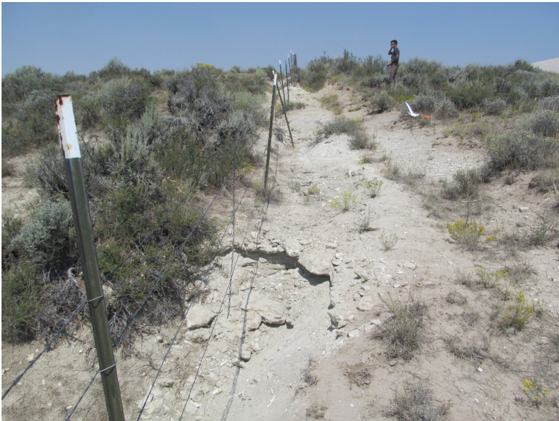
MAW 8/2015. PL-2. Erosion along perimeter fence.
