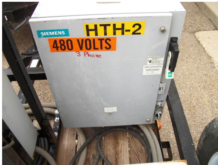
Figure 4. Typical Disconnect Switch
