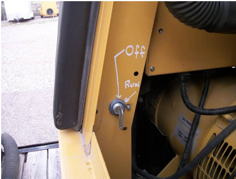
Figure 2. Battery Isolation Switch
