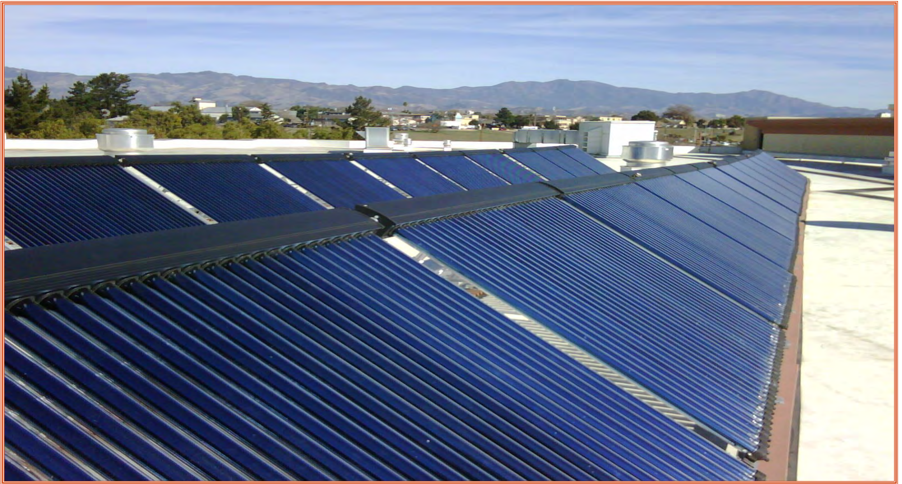
HEAT TRANSFER: Solar Collectors 2011- 720 tubes installed for domestic hot water heating
