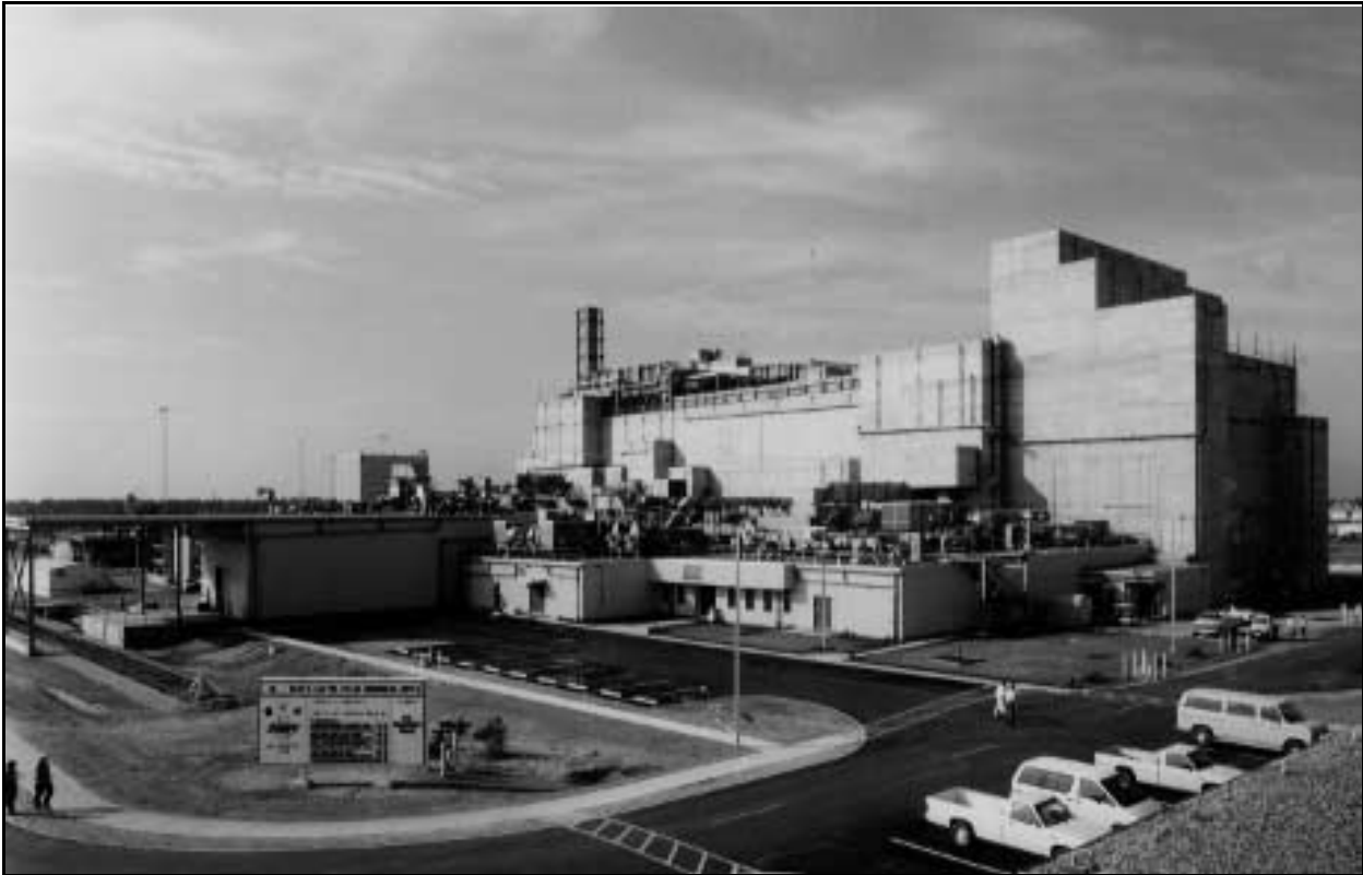
Figure 2–21 Defense Waste Processing Facility at SRS
