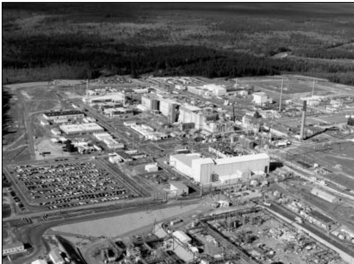
Figure 2–18 The F-Canyon Complex at SRS
