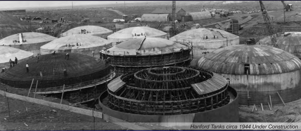
Hanford Tanks circa 1944 Under Construction
