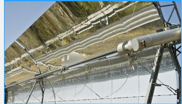
Concentrated Solar Power
