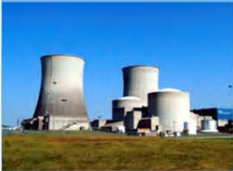
Watts Bar Nuclear Plant
