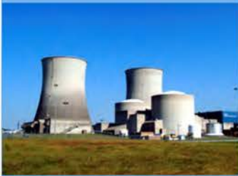
Watts Bar Nuclear Plant
