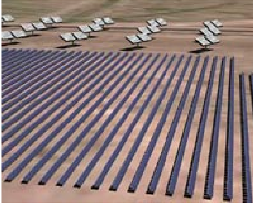
Solar PV Power Plant in Southern Colorado
