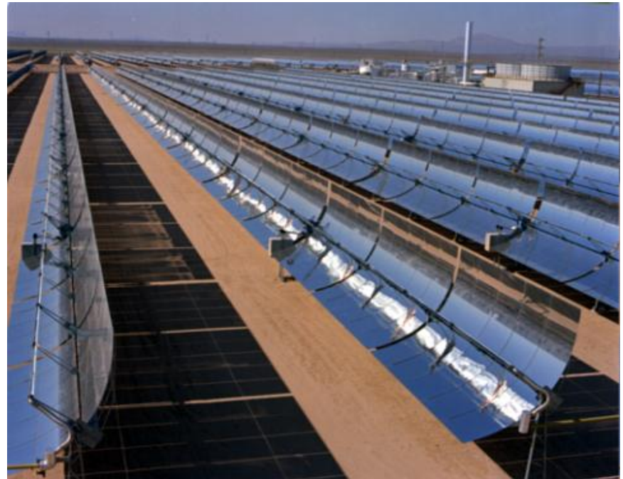
Solar Thermal Power Plant in southern California
