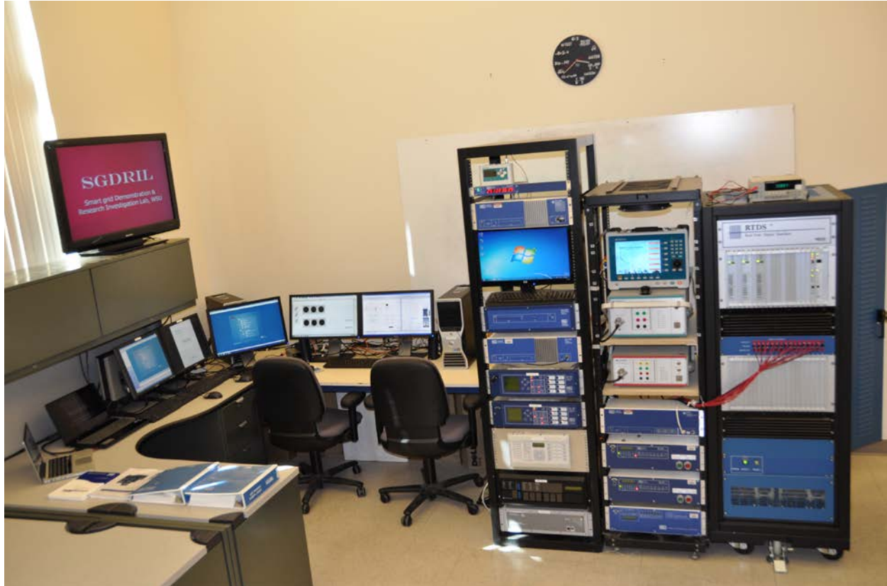
Figure 1: Real time smart grid test bed at WSU
