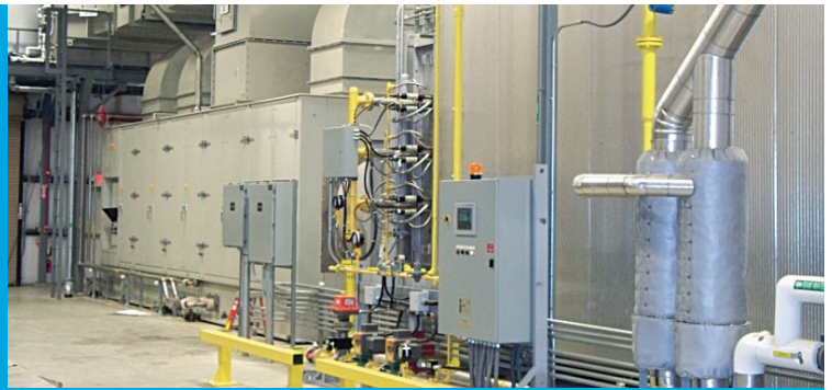
CHP System at Frito Lay facility in Killingly, Connecticut. Photo courtesy of Energy Solutions Center.
