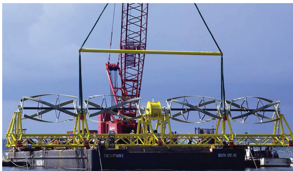
Ocean Renewable Power Company's TidGen™ converts ocean and river currents into clean renewable electricity. Photo from Ocean Power Technologies, NREL 24507
