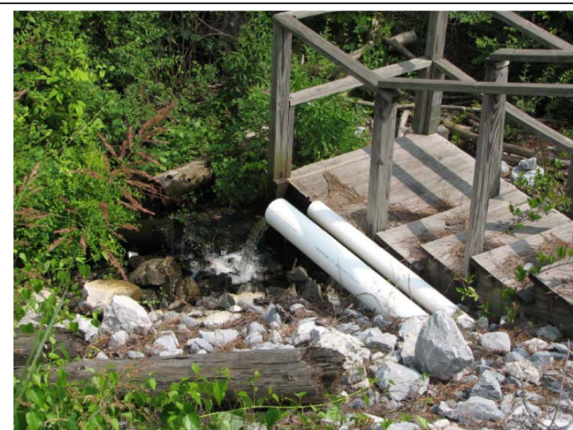
Figure 3-3. Discharge to Railroad Ditch
