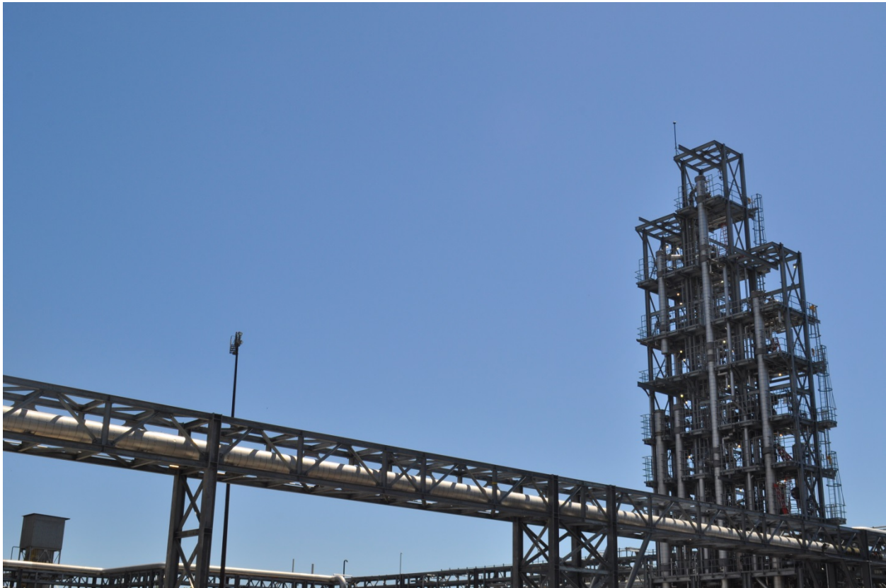
Figure 2-2. Post-Combustion CO 2 Capture Center
