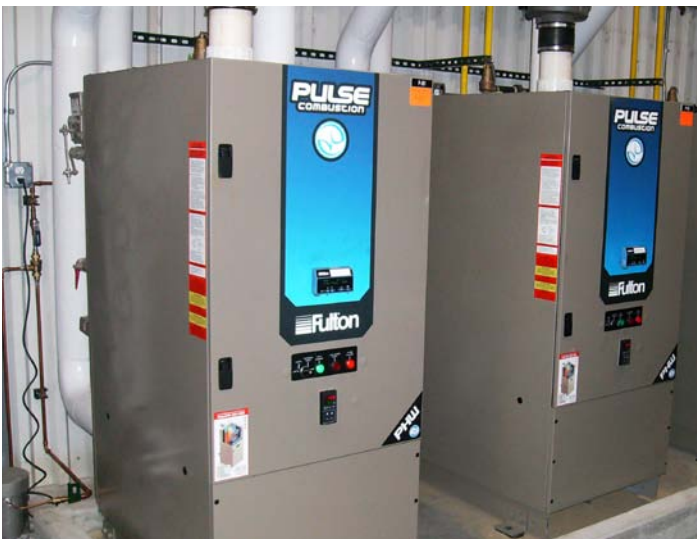
The Briggs & Stratton Wauwatosa, Wisconsin, facility's new steam and heat boiler system.
