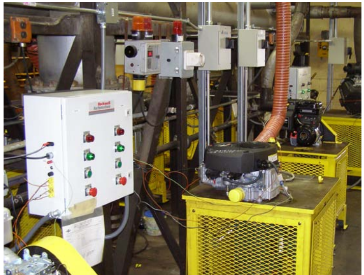
The Briggs & Stratton Milwaukee, Wisconsin, facility's new engine power regeneration system.
