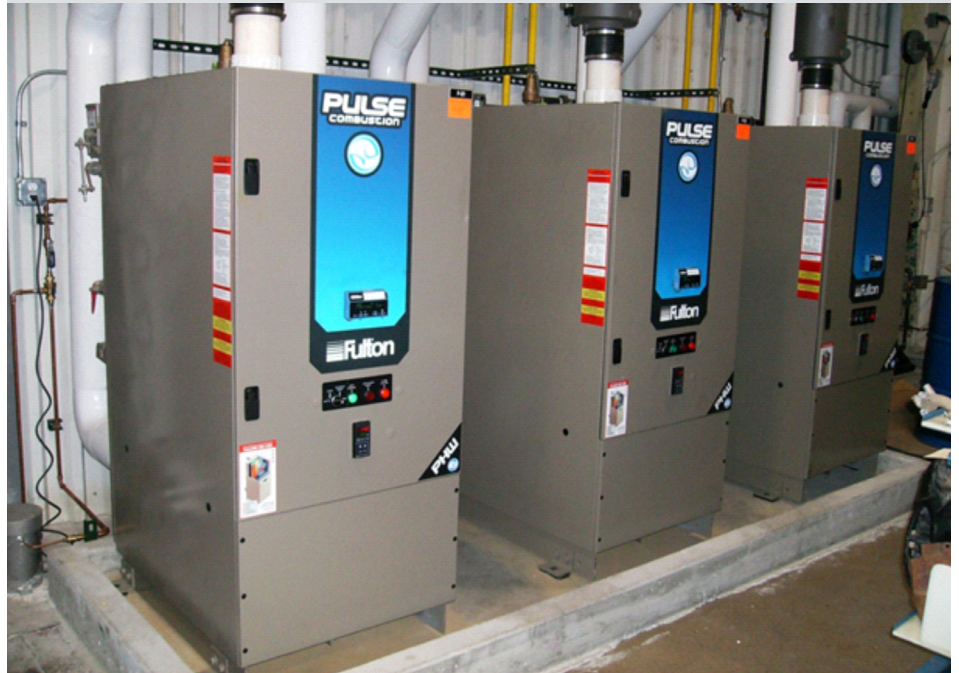
Briggs and Stratton Corporation replaced high-pressure steam boilers with a combination of more efficient low-pressure steam boilers and hot water boilers at its engine manufacturing facility in Wauwatosa, Wisconsin. Photos courtesy of Briggs and Stratton Corporation
