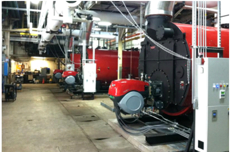
Briggs and Stratton Corporation replaced high-pressure steam boilers with a combination of more efficient low-pressure steam boilers and hot water boilers at its engine manufacturing facility in Wauwatosa, Wisconsin. Photos courtesy of Briggs and Stratton Corporation
