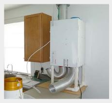
An energy recovery ventilator was modified to provide mechanical ventilation in a supply-only mode, with no heat or enthalpy recovery.
