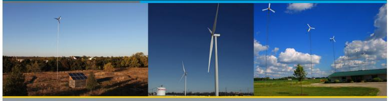
The distributed wind market includes wind turbines and projects of many sizes, such as a Pika T701 1.80-kW wind turbine paired with a 2-kW solar array in Kansas, two GE 1.7-MW wind turbines at a Honda transmission plant in Ohio, and six Bergey Excel-S 10-kW wind turbines in Ohio. *Photos from left to right: from Kelsey Kaufman; from Honda.com; from Mark Spears.*
