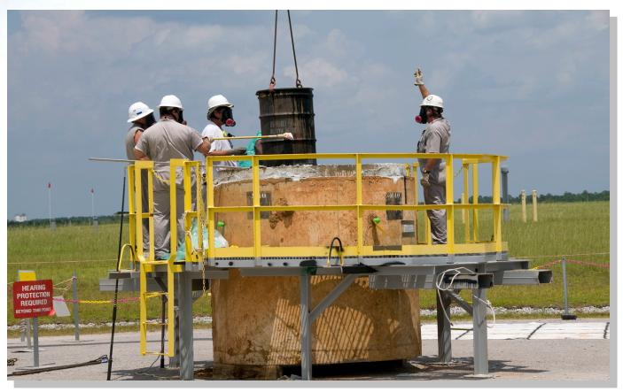
TRU waste drums being removed from a concrete culvert
