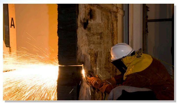
A shield door is being cut in preparation for D&D activities in P Reactor
