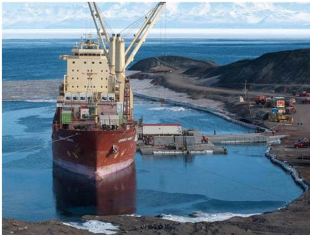
Figure 25. Modular causeway system used by the U.S. Army
