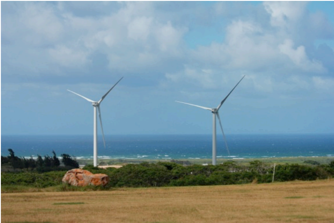
Figure 1. Oahu's Kahuku wind power plant
