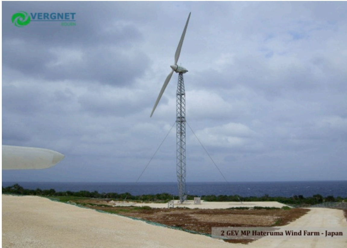
Figure 20. Vergnet MP C turbine
