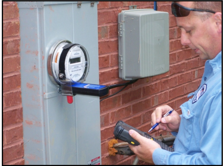
A Tri-State technician checks a newly installed next-generation smart meter.
