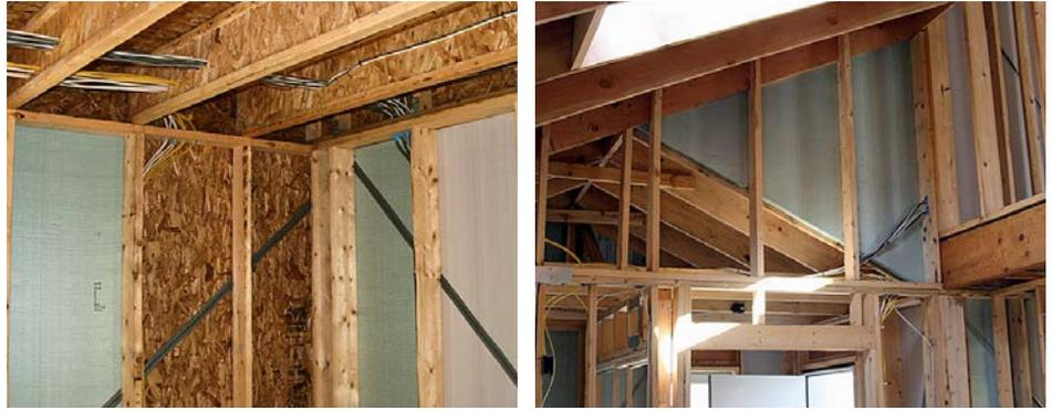
Advanced framing techniques such as two-stud corners and stacked framing (above left) save labor and materials, but they also simplify the installation of spray foam insulation and reduce the number of air leakage paths. However, complex framing to create architectural details (above right) needs to be considered carefully in order to ensure continuity of the air barrier system.
