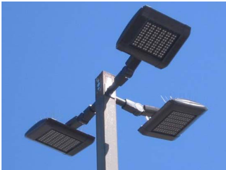
Close up view of new LED luminaires atop an existing light pole.
