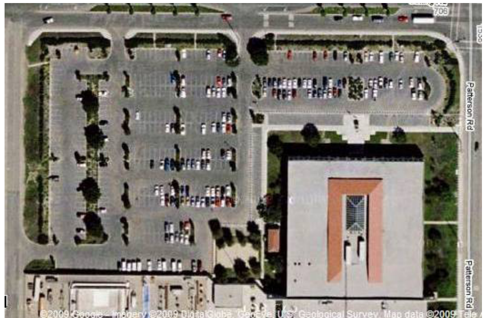
The parking area around building 1100 is fairly typical. The parking area wraps part-way around the building. There are some scattered trees, shrubs and other vegetation planted in the medians. The parking area is illuminated by lights atop 12, 33-1/2-foot square poles.
