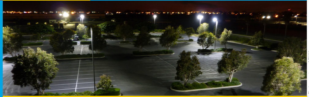
New LED parking area lights at the NAVFAC Engineering Service Center at Port Hueneme provide high quality, evenly distributed light.
