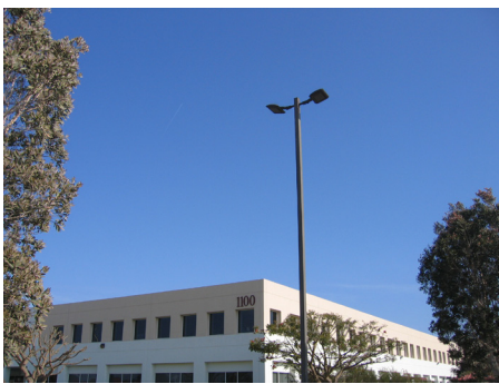
New LED lights over the parking area.
