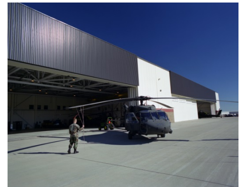
SVP Installed System
