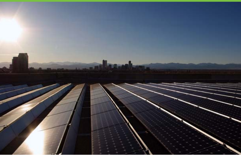
This PV array has 465 solar panels split between roofs on the southeast and southwest wings of the Denver Museum of Nature and Science. The installation was made possible through a collaboration of Hybrid Energy Group, Partnership for Sustainability, Xcel Energy, and Namaste Solar Electric. Photo from Denver Museum of Nature and Science, NREL/PIX 18045
