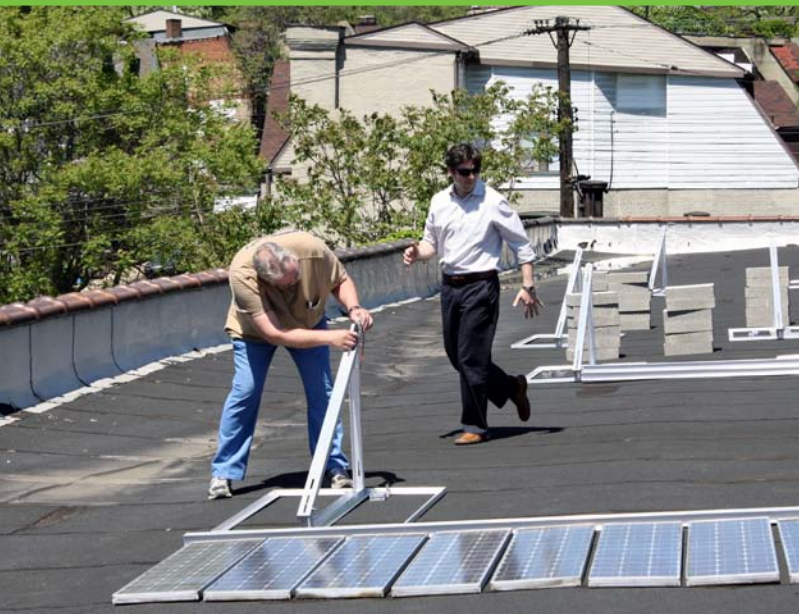
Solar professionals make progress on a PV array on Pittsburgh's public works garage. Photo from City of Pittsburgh, NREL/PIX 18414
