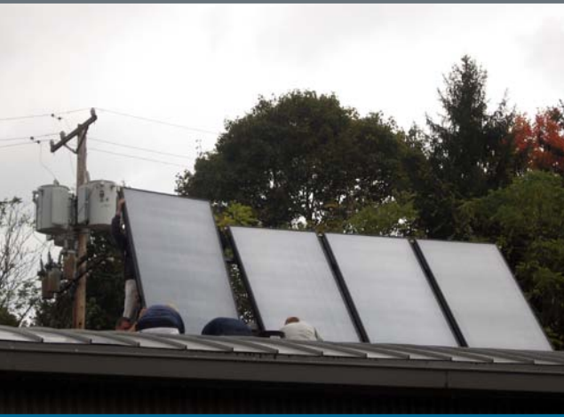
An installer puts a solar hot water system on Pittsburgh Truck House No. 34. Photo from City of Pittsburgh, NREL/PIX18412
