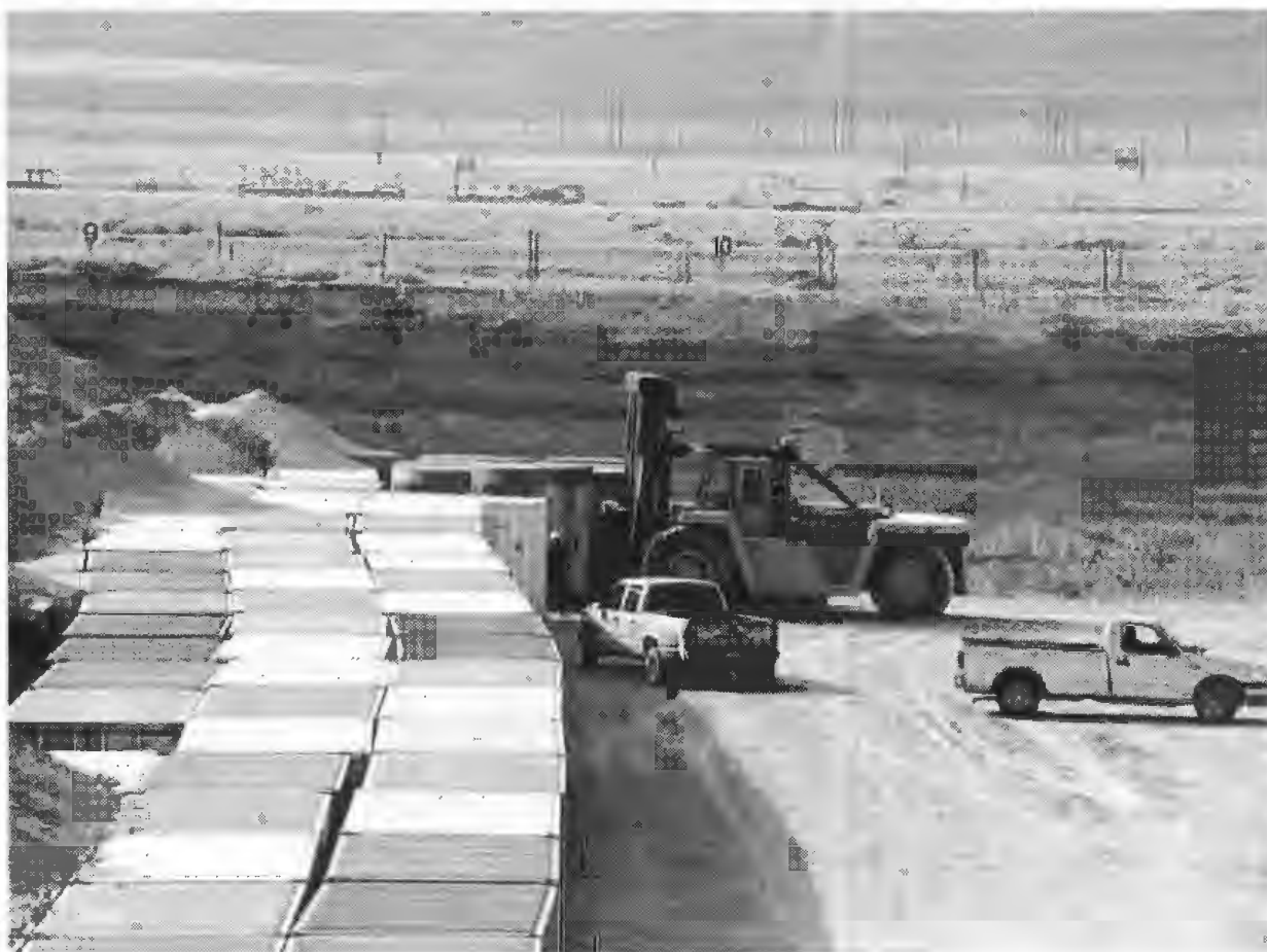
Area 3 Radioactive Waste Management Site Concrete Monolith of Low-Level Waste Disposed in Area 3, Nevada National Security Site
