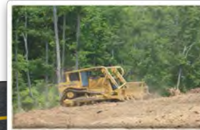
2012: Expansion of onsite disposal facility complete
