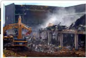
2006: Building K-29 at ETPP demolished
