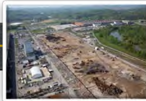
2010: Building K-25 West Wing demolished
