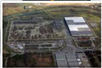
2011: Building K-33 at ETPP demolished
