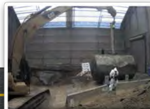
2012: Tank W-1A at ORNL removed
