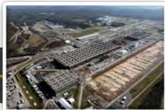
2011: Building K-25 East Wing demo begins
