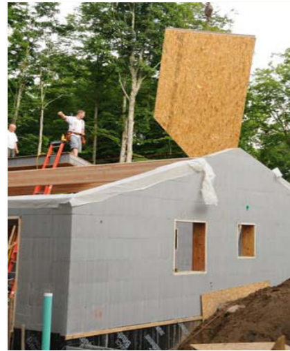
Figure 5. Construction with SIPs
