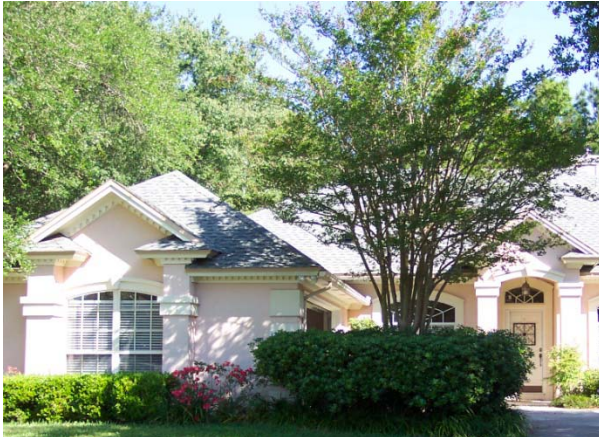
House 1: Buried & Encapsulated
