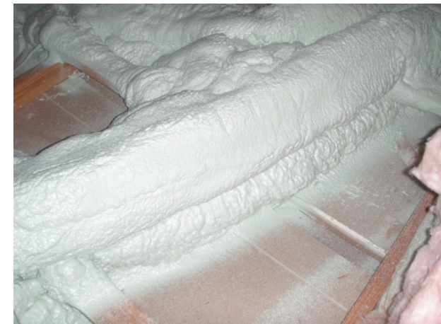
Well-sealed ductwork
