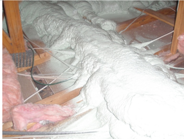
Existing flues must be protected
