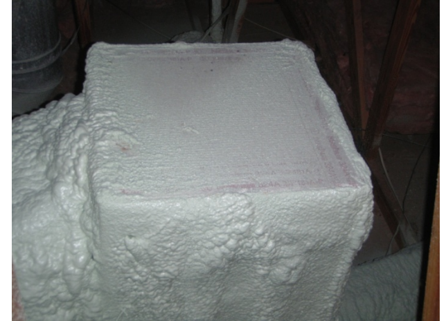
Supply plenum box inadequately spray foamed
