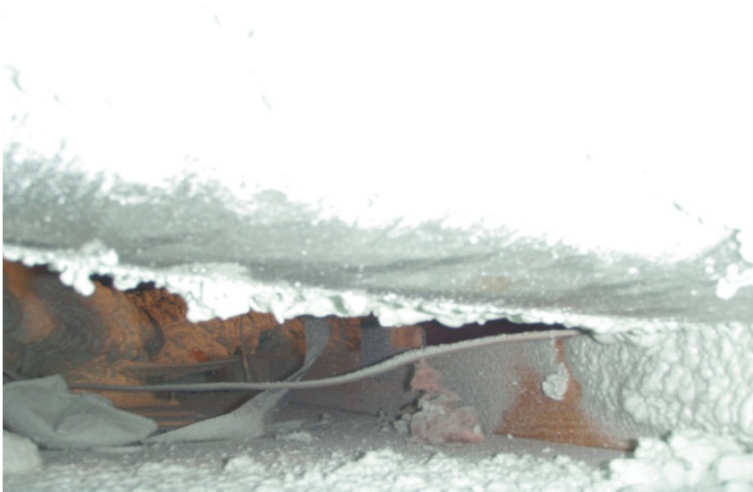
Exposed underside of duct
