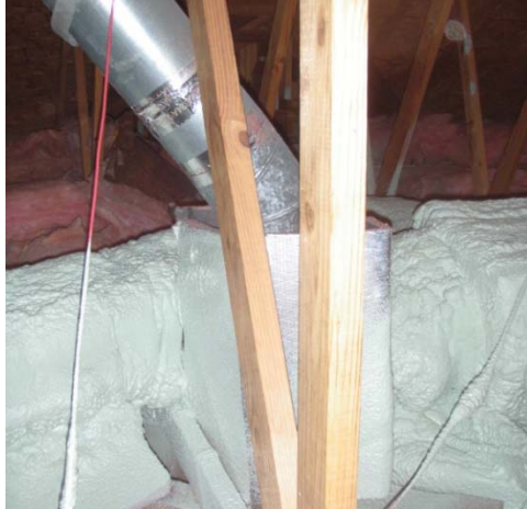
Existing flues must be protected
