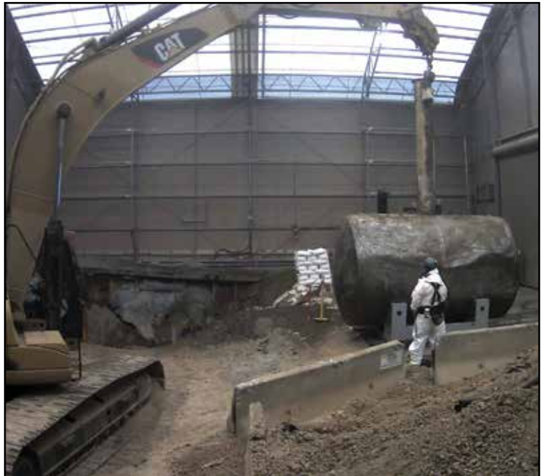
Removal of Tank W-1A at ORNL
