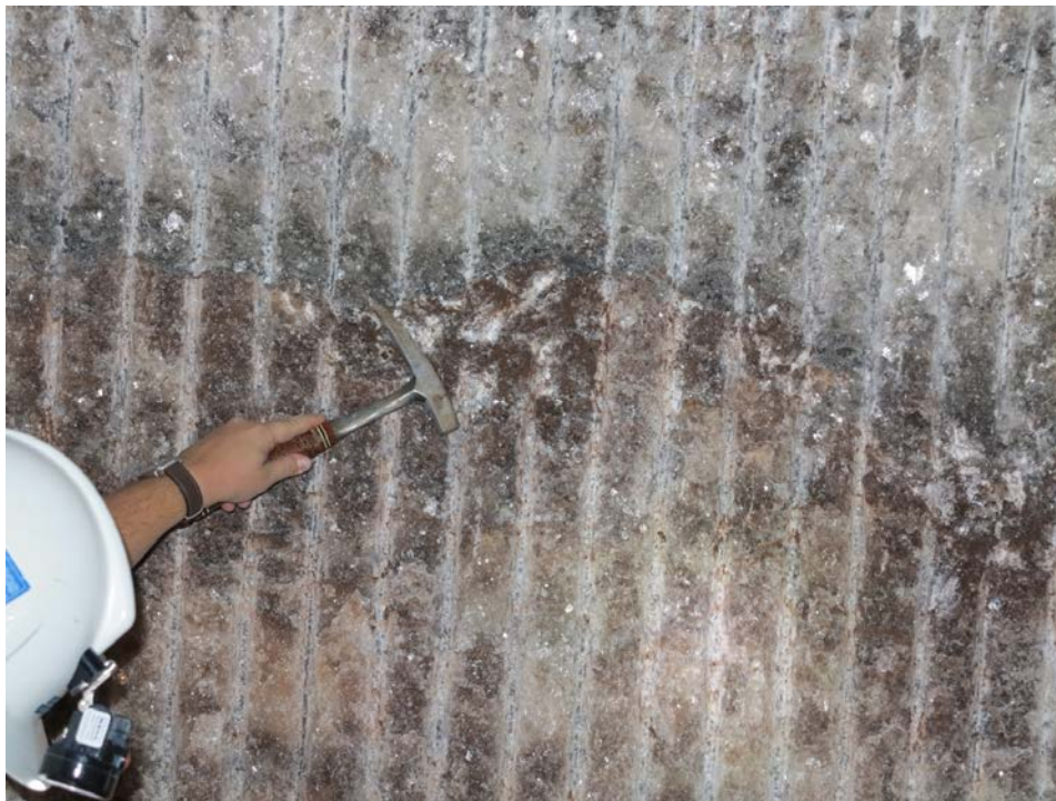
Figure 4. Picture of the clay rich zone in orange marker bed in the newly excavated SDI rooms E690N500-N350.
