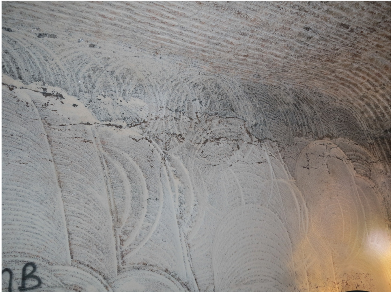
Figure 3. Picture of the clay (corrensite) seam F in the newly excavated SDI rooms E690N500-N350.
