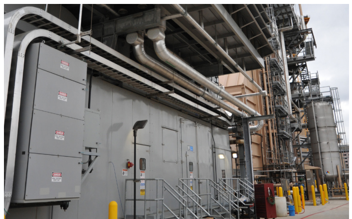
Thermal Energy Corporation installed a natural-gas fired CHP system at the Texas Medical Center in 2010.
