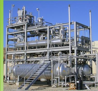
DOE Small Business Innovation Research (SBIR) support enabled TDA to develop and commercialize its direct oxidation process—a simple, catalyst-based system for removing sulfur from natural gas and petroleum—that was convenient and economical enough for smaller fuel processing plants to use.
