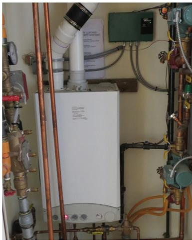
A wall-hung condensing boiler with an efficiency rating of 92.5 AFUE provides hot water for domestic use and for radiant floor heating.
