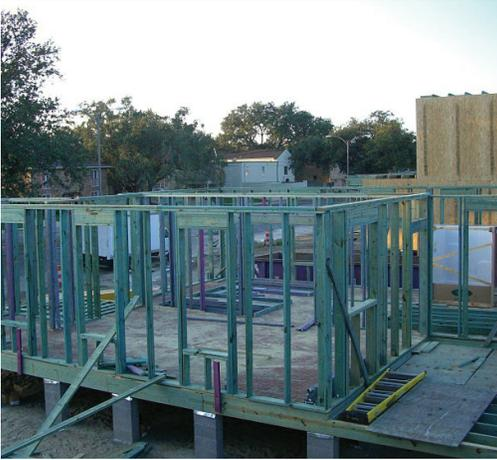
Advanced framing techniques including 2x6, 24-inch-on-center stud walls to reduce lumber use and thermal bridging. All framing was made of borate pressure-treated lumber, rendering it extremely termite, mold, and mildew resistant.
