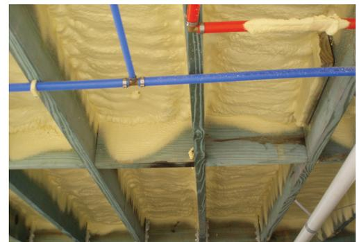
(top) Building America’s Building Science Consortium team recommended insulating the attics with high-density closed-cell spray foam, which gives excellent air sealing and thermal performance while providing conditioned space for the high-efficiency HVAC equipment and ducts (Courtesy of Green Coast Enterprises)
