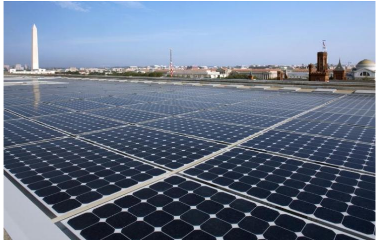
DOE HQ solar array on the roof of the Forrestal North Building
