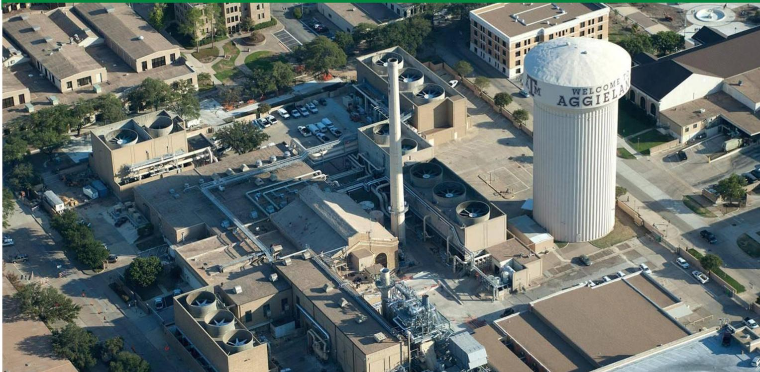
The CHP system at Texas A&M is now capable of producing 50 MW of on-site generation.
