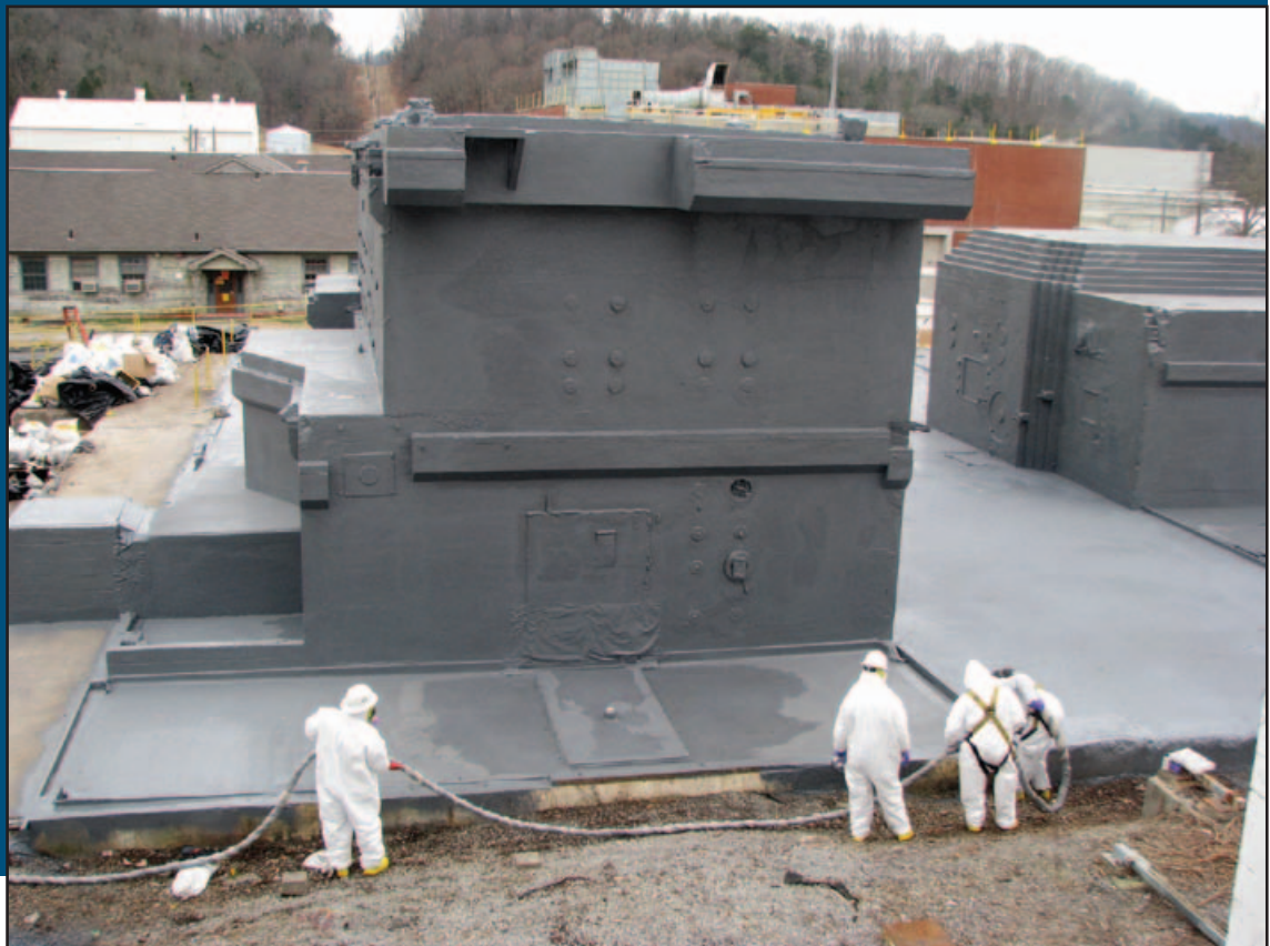
Remaining hot cells with polyurea coating
