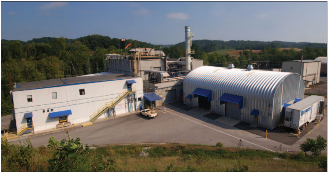
Transuranic Waste Processing Center
