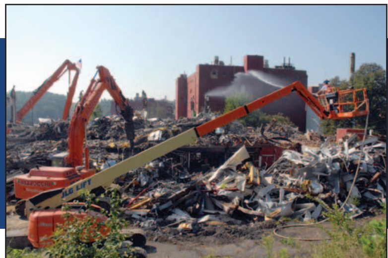
Biology Complex demolition
