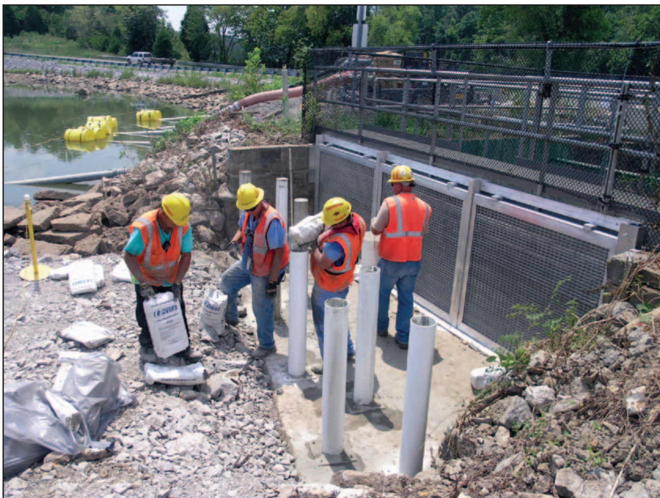
Workers repair a fish barrier at the ETTP P1 Pond to prevent fish from migrating into the pond from Poplar Creek
