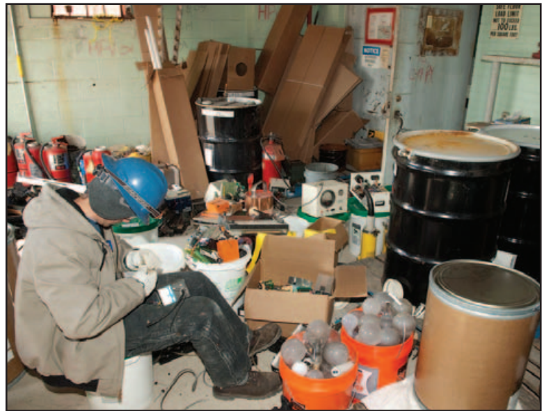
Hazardous material abatement in Building 9220, part of the Biology Complex
