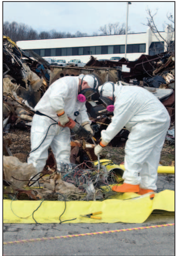
Workers cut materials for samples
