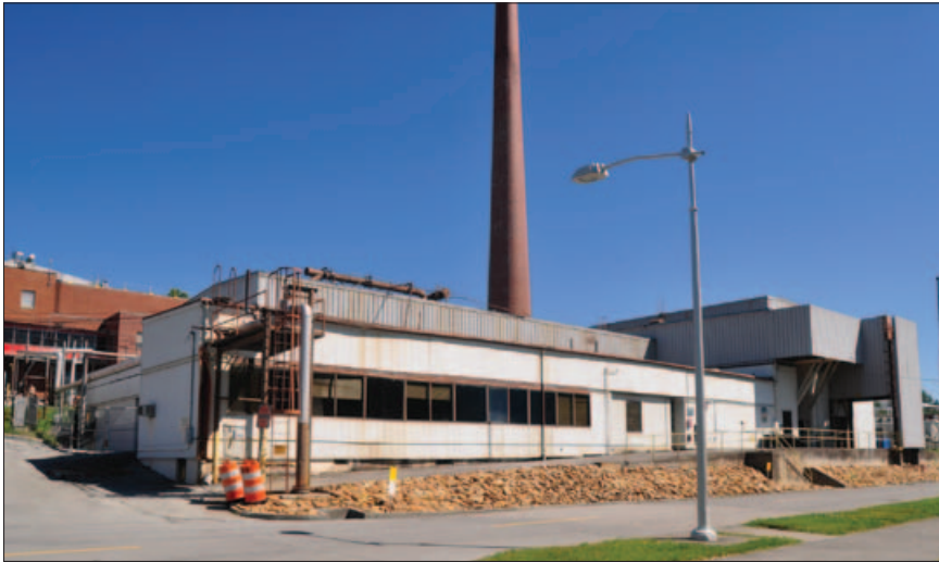
3026 facility before demolition
