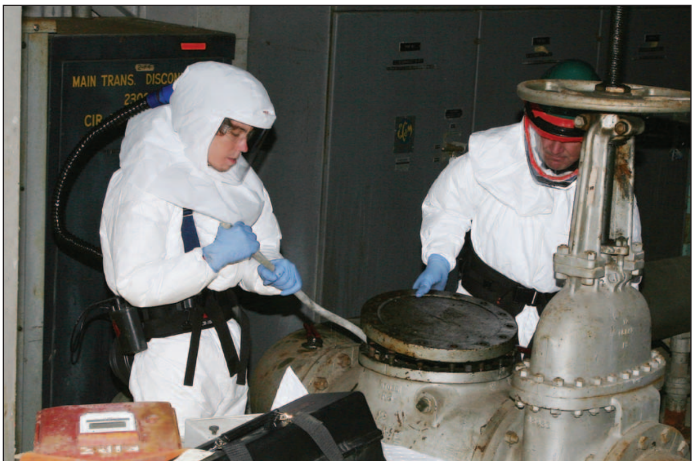
Workers open a cooling water pump system in preparation for characterizing the waste in Building 3103, one of the 34 non-reactor facilities to be demolished
