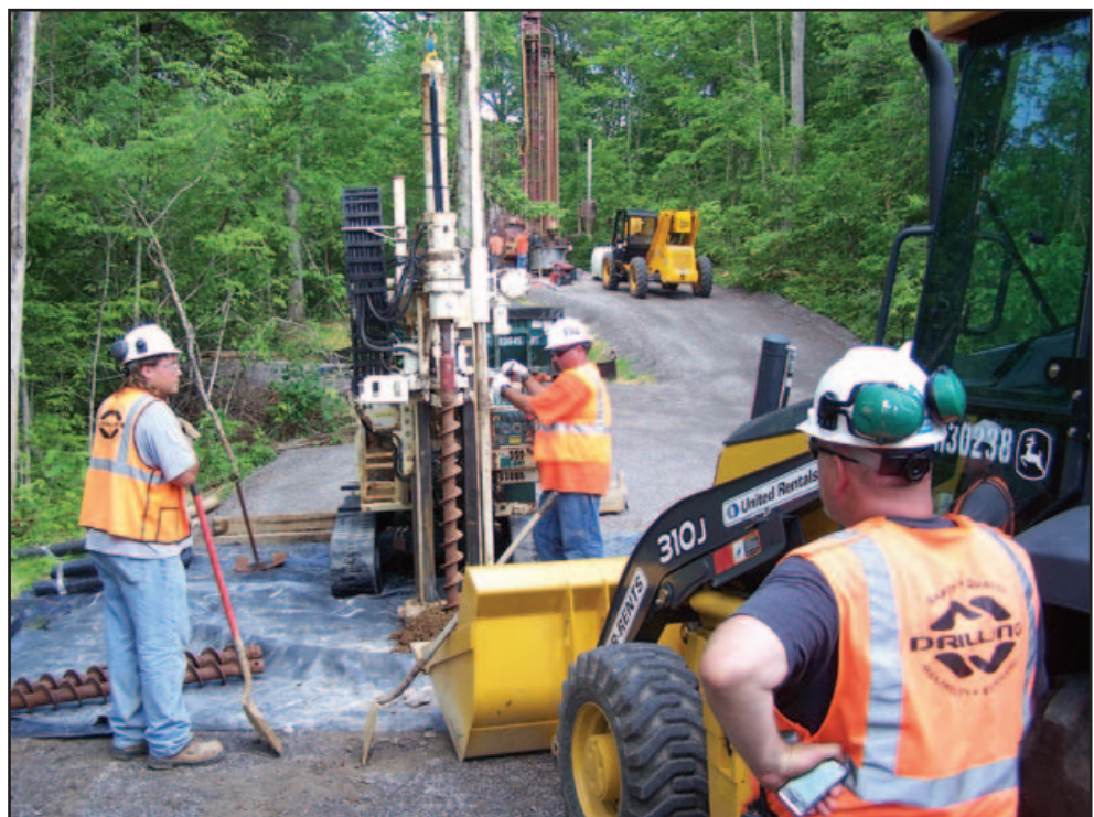
Workers are installing one of three new monitoring wells along Raccoon Creek
