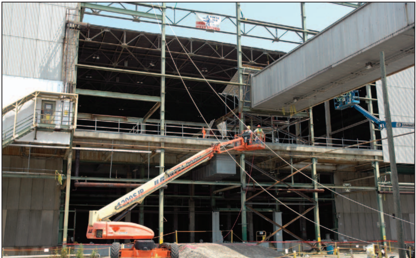
Workers complete the final steps in isolating the tie line that connected the K-33 Building to the K-31 Building
