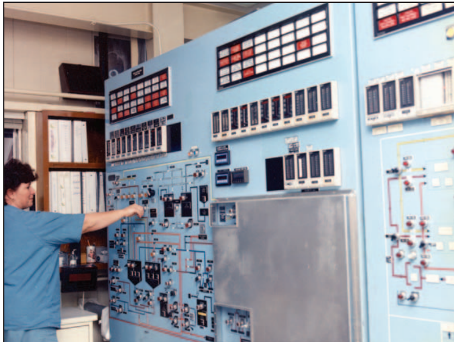
Central Neutralization Facility control room
