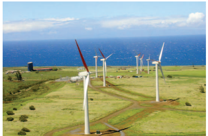
Courtesy of Hawaiian Electric Light Company (HELCO)
