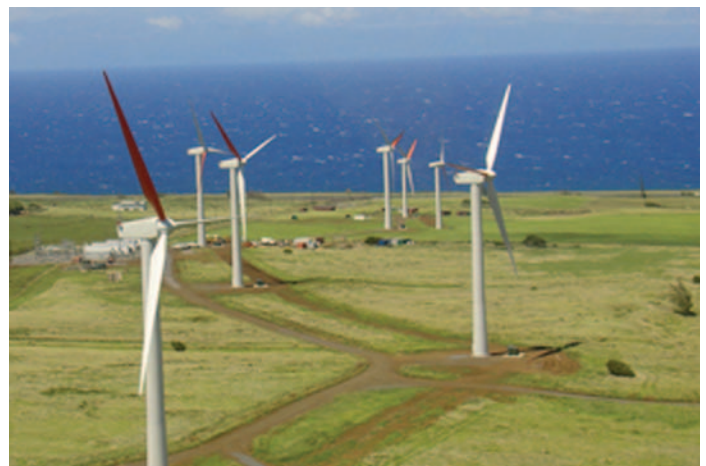
Courtesy of Hawaiian Electric Light Company (HELCO)
